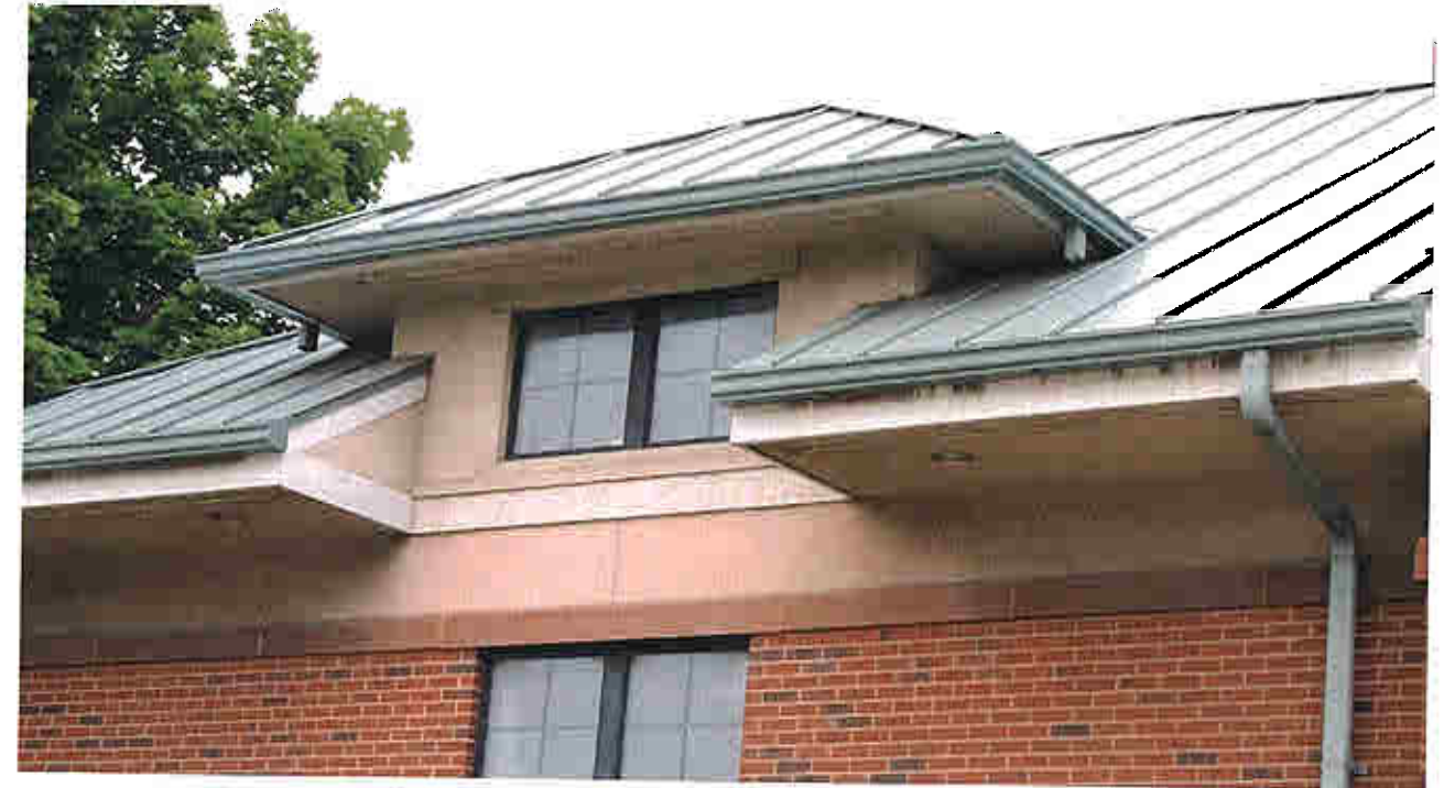
Standing Seam Metal Roof
