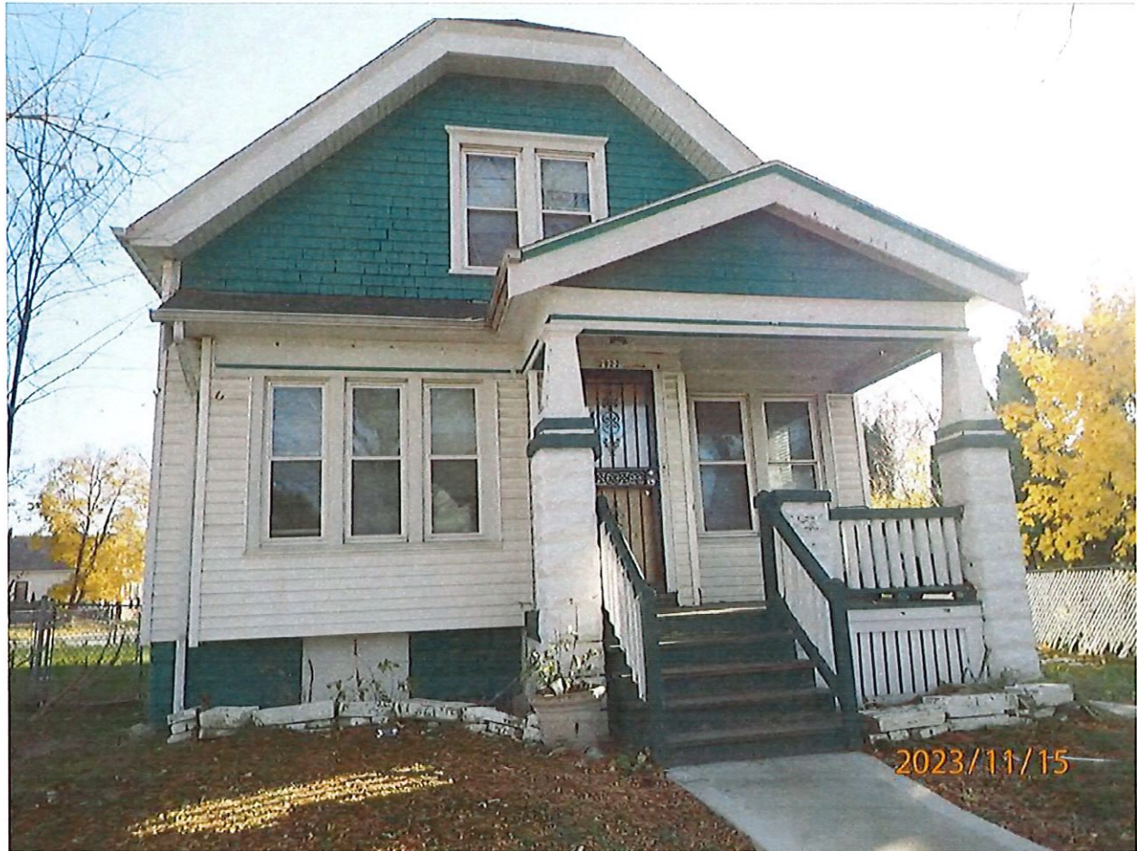
Above: Photo of the Subject Property (2922 North 16 th Street)
