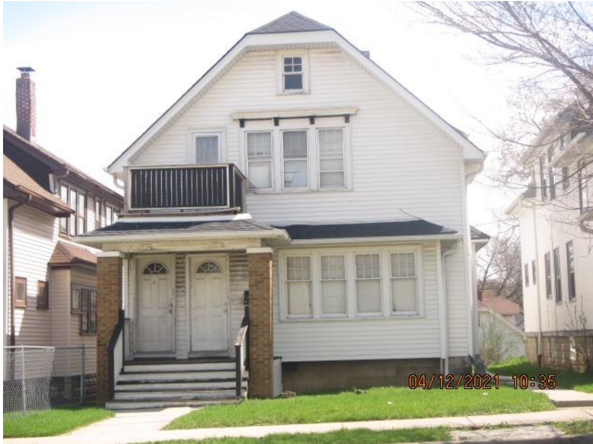
3532-34 North Port Washington Ave
