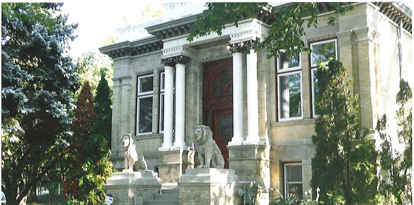
VIEW LOOKING SOUTHEAST AT THE LION HOUSE FROM WEST HIGHLAND BOULEVARD
