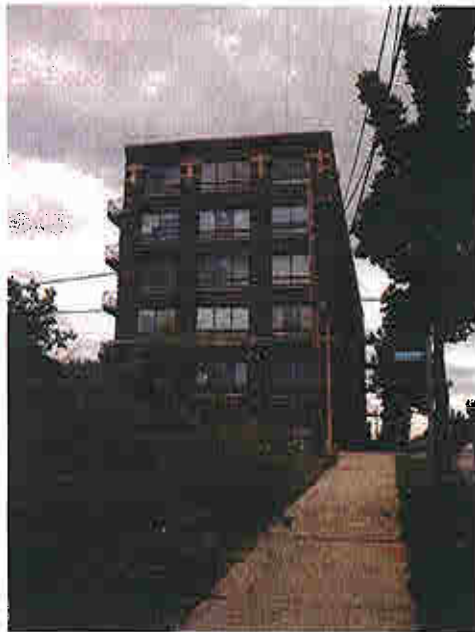
6. 234 E RESERVOIR AVE
