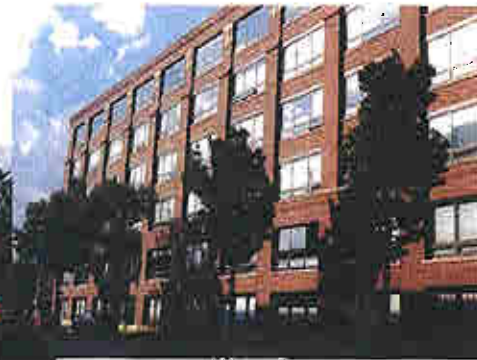
10. 234 E RESERVOIR AVE
