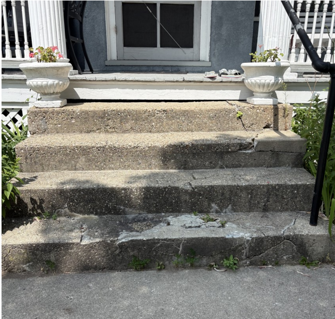
Front steps to be replaced, railing reused.
