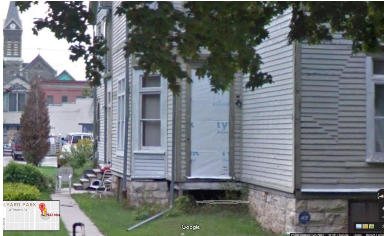
Current conditions showing current stairs that do not meet code.
