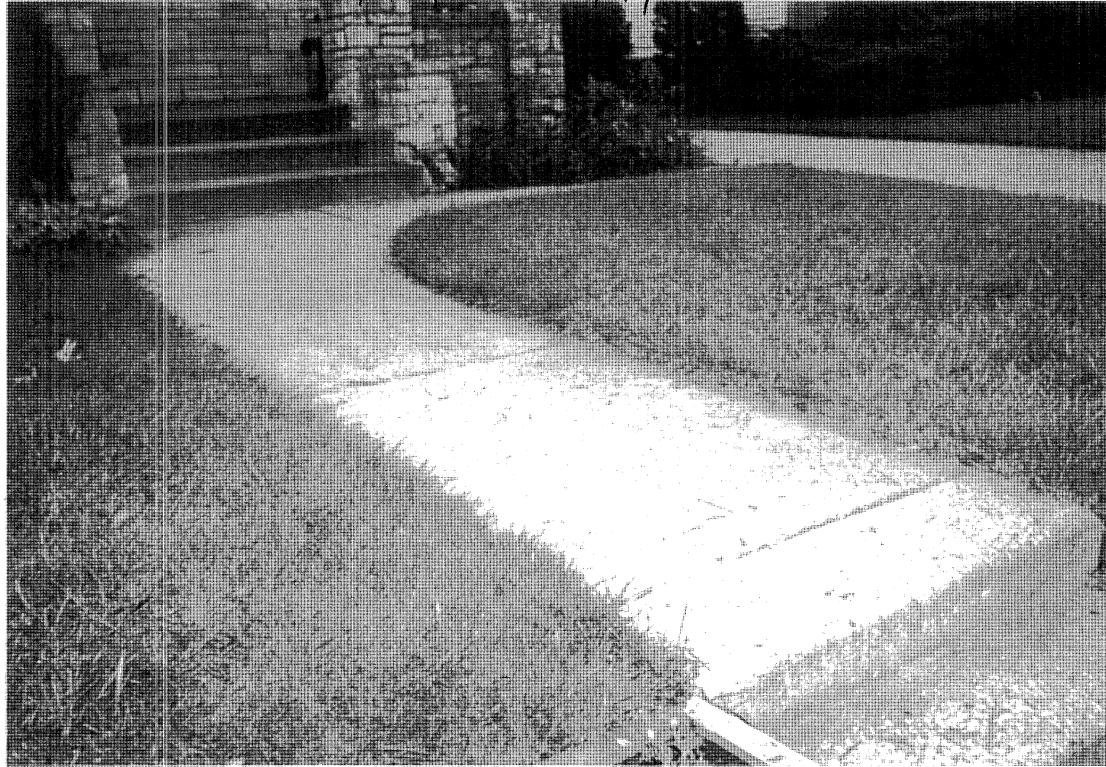
END OF Collapsed Pipe
