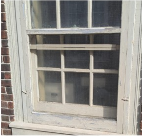
Window missing storm window, with vinyl plastic visible from exterior, as well as remnants of the closing swivels from original storm window
