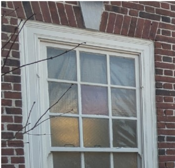
Window missing storm window, with vinyl plastic visible from exterior, as well as remnants of the closing swivels from original storm window
