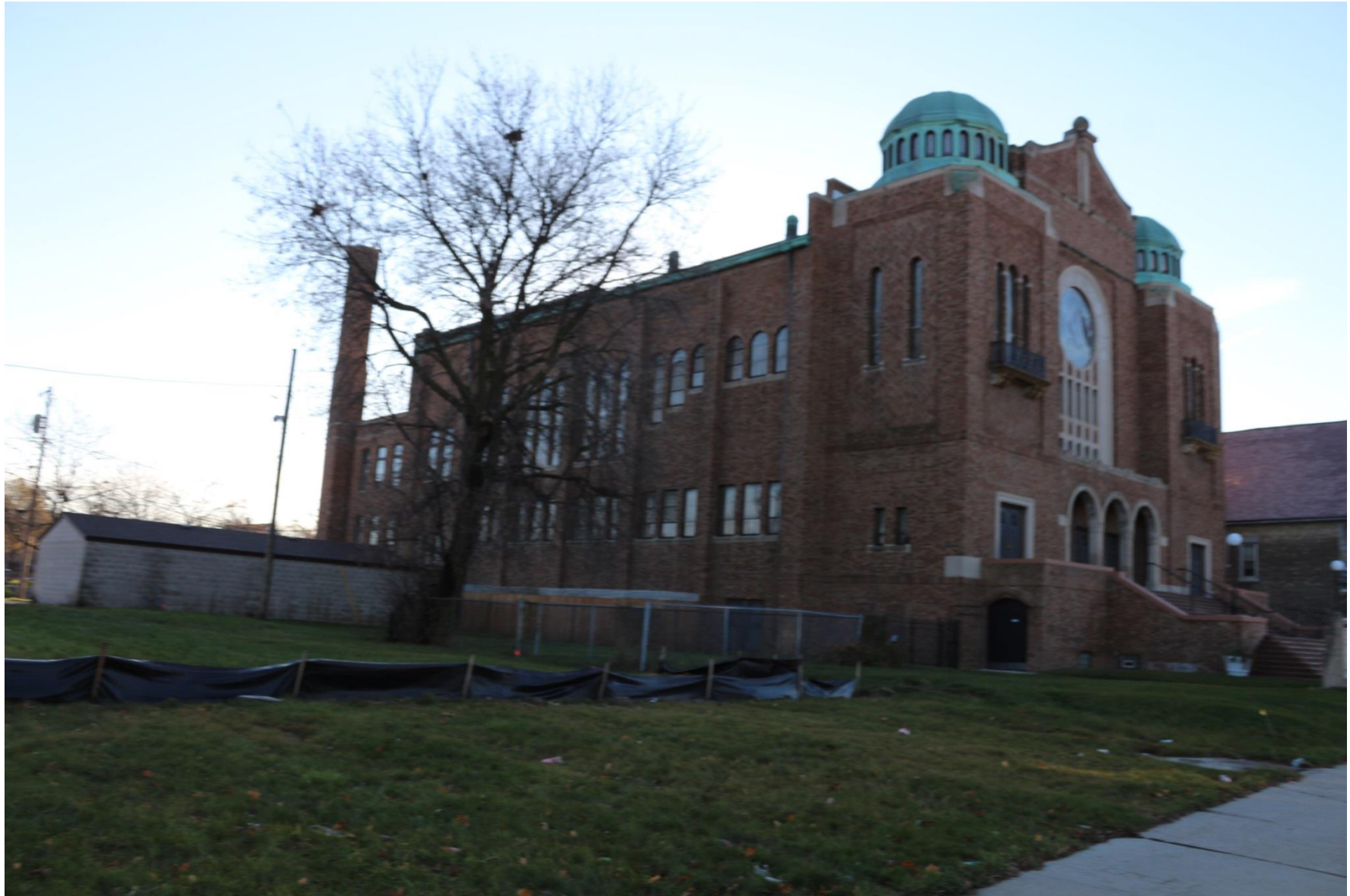
Existing conditions, looking south along Teutonia. Garage at rear (left) is to be demolished.
