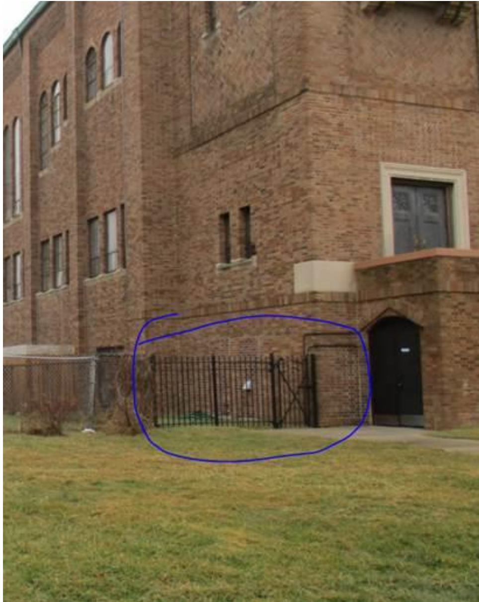
Fencing to be duplicated and extended across courtyard
