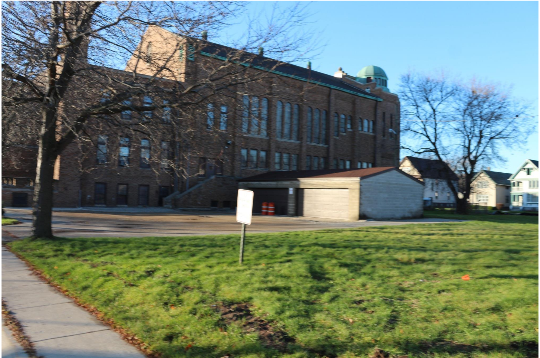
North elevation where connector will be attached. Garage will be demolished.
