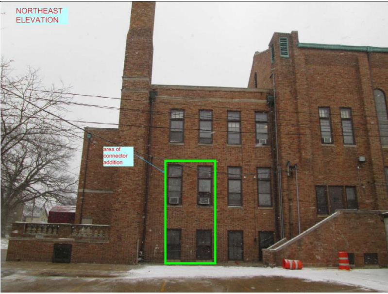
Point of connection. These 4 windows will be removed.
