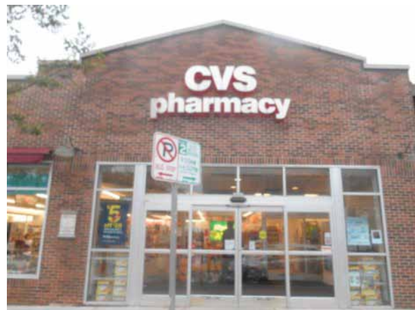
Remove Existing Letters (Patch Holes)
