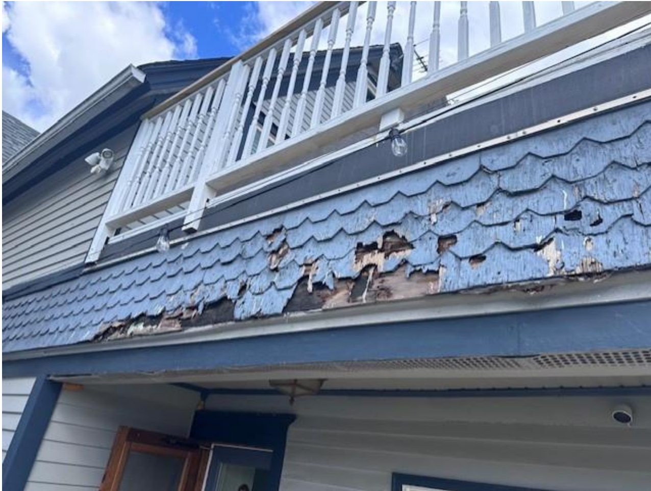
Existing cedar siding to be replaced in-kind
