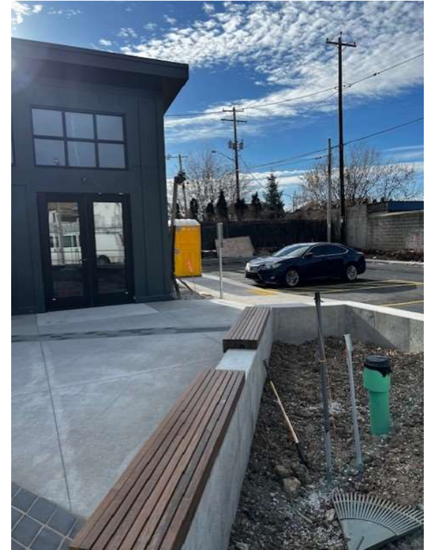
Concrete pavers and seating units
