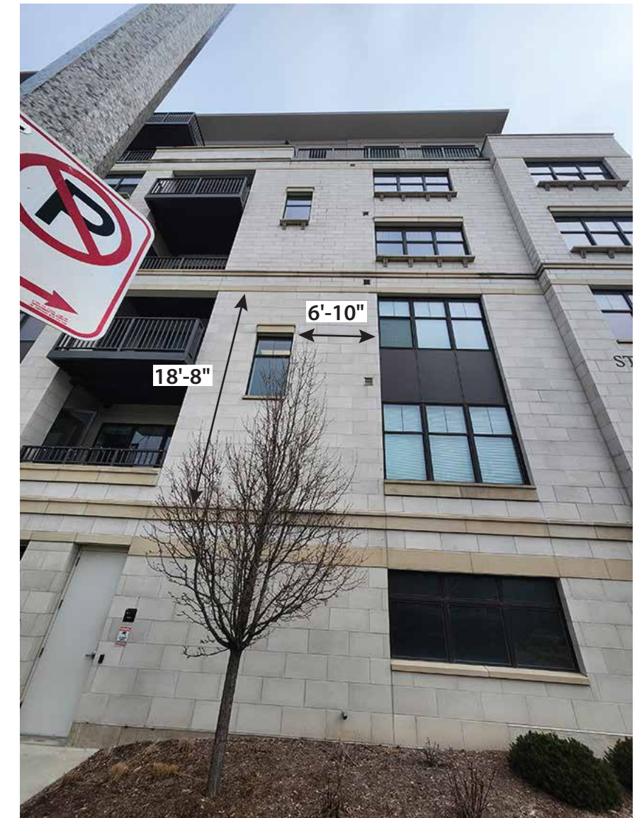
Building Dimensions: From the top of the window to the concrete bump out is 18'-8" H and 6'-10" W is the space between the windows. Center sign vertically & horizontally in that area.
