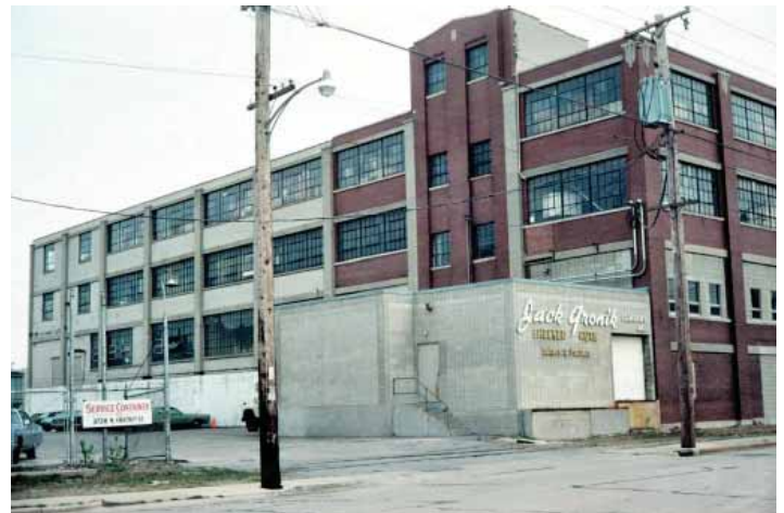
Figure 1.9 Older industrial building in Riverworks Source: City of Milwaukee, Department of City Development
