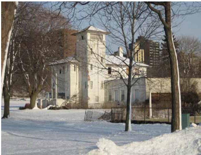
Figure 11.33: Former Coast Guard Station Slated for Demolition
