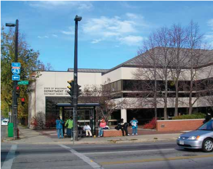
Figure 5.32: DNR Building and site to be Redeveloped
