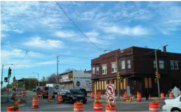
Figure 7.25: Center Street and Holton Street - Existing Conditions
