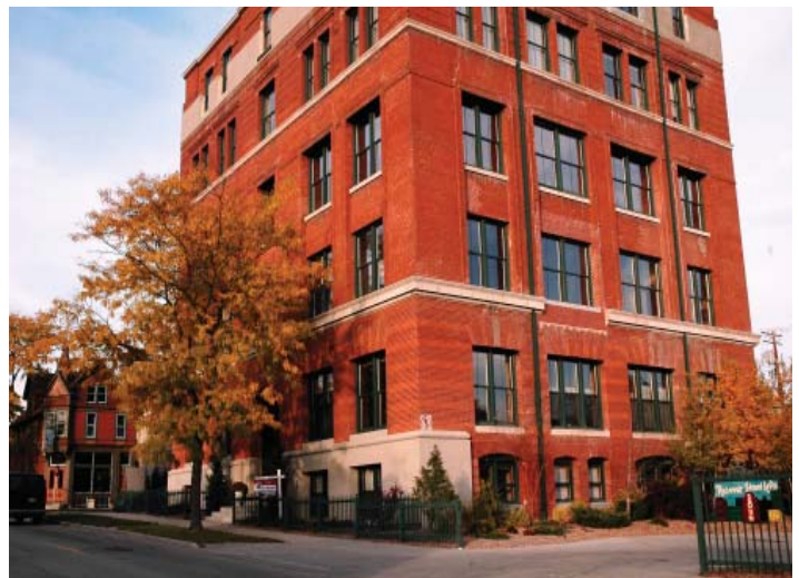
Figure 2.25: Reservoir Street Lofts
