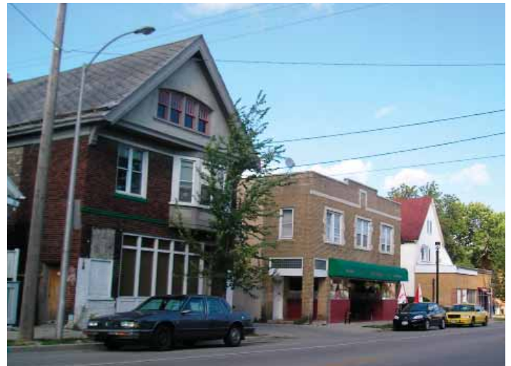
Figure 7.16: Center Street - Existing Streetscape Conditions
