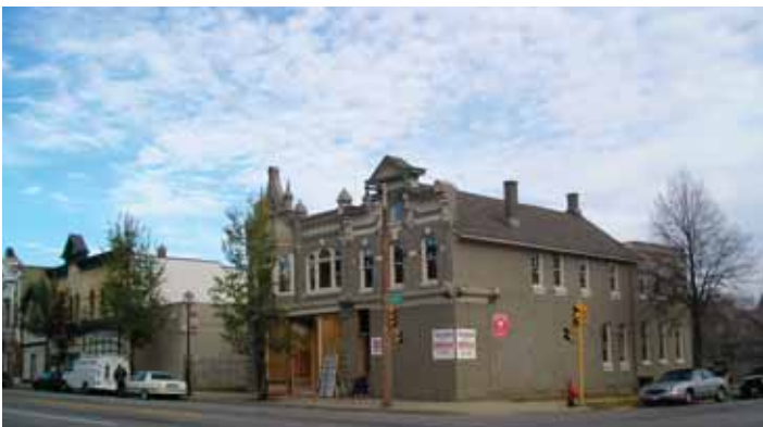
Figure 7.26: Center Street and Holton Street - Existing Conditions
