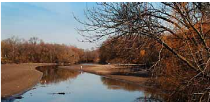
Figure 8.16: Floodplain created by North Avenue Dam removal.
