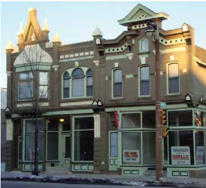
Figure 5.34: Historic Building after facade renovation.
