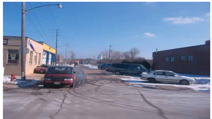
Figure 6.3: Existing Roadway Conditions
