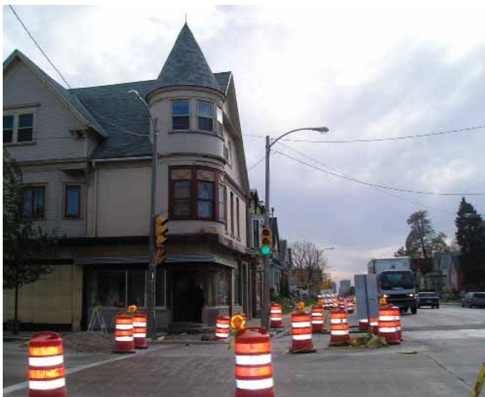
Figure 7.21: Holton Street - Existing Streetscape Conditions
