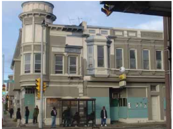
Figure 5.39: King Drive and Center Street Existing conditions
