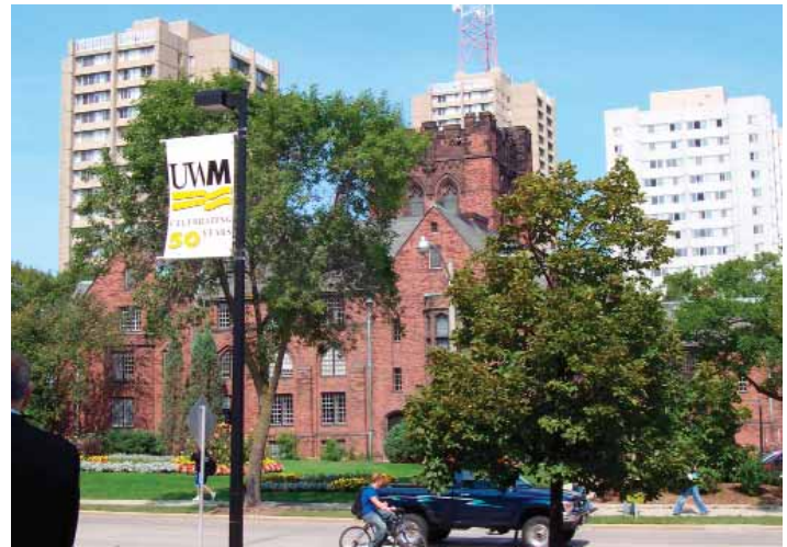
Figure 3.16: UWM: Chapman Hall
