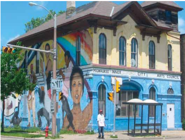
Figure 5.7: Former Milwaukee Inner City Arts Council building
