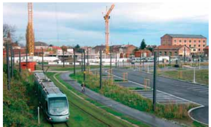
Tramway in Valenciennes. The urban landscape associated with the tramway can be used to increase the value of the areas through which they run: paving materials can be changed, trees can be planted and grass can be laid along the tramway tracks.
