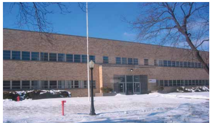
Figure 6.4: Existing Industrial Buildings
