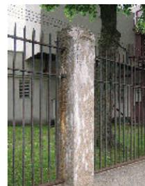
**Figure 15.** Evidence of moisture movement through concrete is apparent in the form of mineral deposits on the concrete surface. Cyclic freezing and thawing of entrapped moisture, and corrosion of embedded reinforcement, have also contributed to deterioration of the concrete column on this fence at Crocker Field in Fitchburg, Massachusetts, designed by the Olmsted Brothers.
