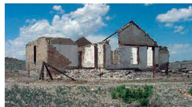
**Figure 2.** Chatterton House was the home of the post trader at Fort Fred Steele in Wyoming, one of several forts established in the 1860s to protect the Union Pacific Railroad. The walls of the post trader's house were built using stone aggregate and lime, without cement. The use of this material presents special preservation challenges.
