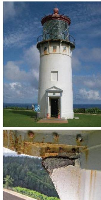
**Figure 12.** The concrete lighthouse at the Kilauea Point Light Station, Kilauea, Kauai, Hawaii, was constructed circa 1913. The concrete, which was a good quality, high strength mix for its day, is in good condition after almost one hundred years in service. Deterioration in the form of spalling related to corrosion of embedded reinforcing steel has occurred primarily in areas of higher ornamentation such as projecting bands and brackets (see close-up photo).
