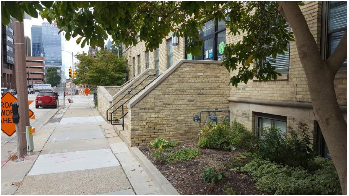
Exhibit C View of east facade of ramp and stair. Existing gas meter to remain.
