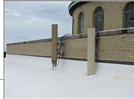
EXISTING T-MOBILE ANTENNAS - GAMMA SECTOR -
