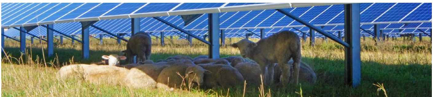
Dairyland Power Cooperative, La Crosse
