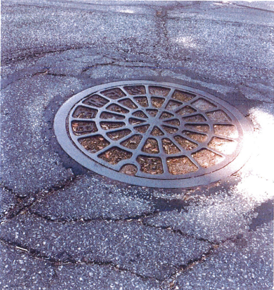
Typical manhole cover installation. Note: no 'lip', cover is sitting flush with street.
