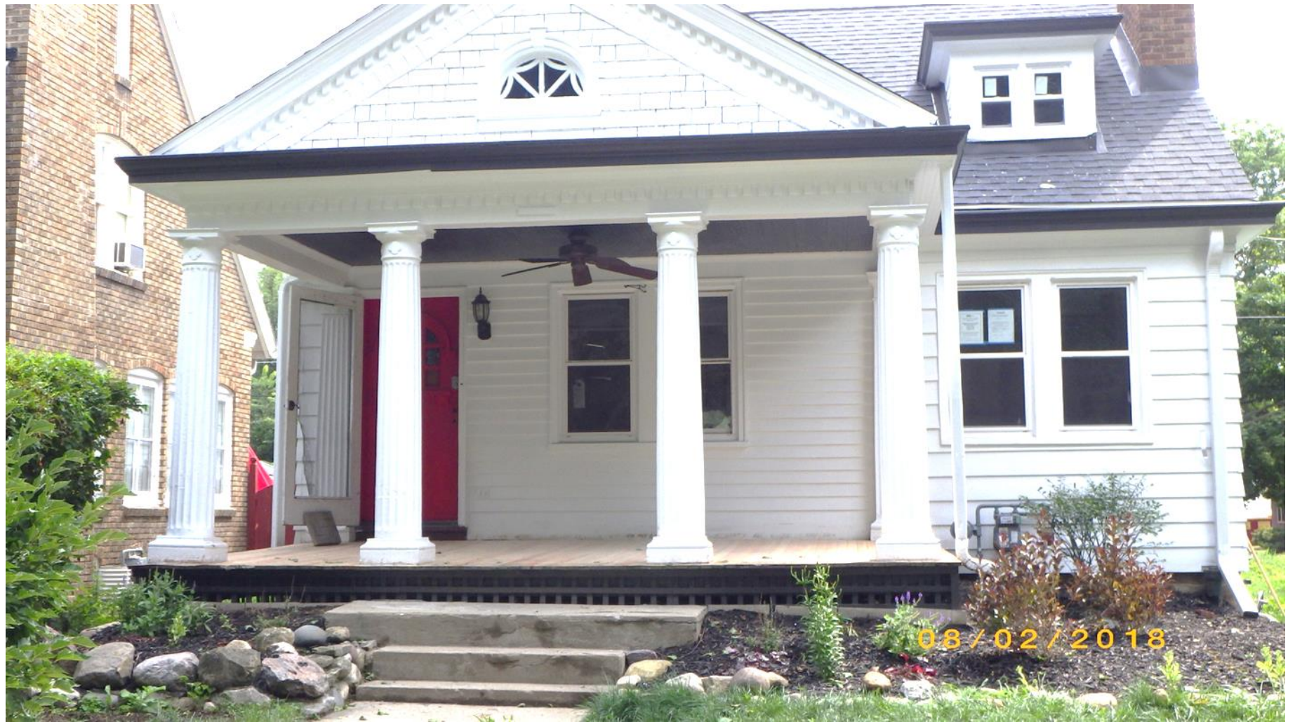
Roof, porch, and siding approved as completed in this photo.
