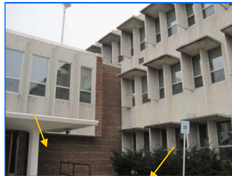
Brick and precast concrete exterior
