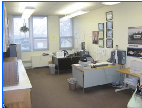
Offices that require paint finishes
