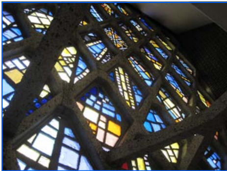
Interior view of mosaic curtain wall
