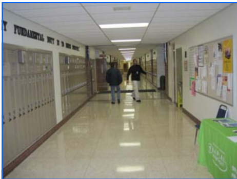
Acoustic ceiling tile in hallway
