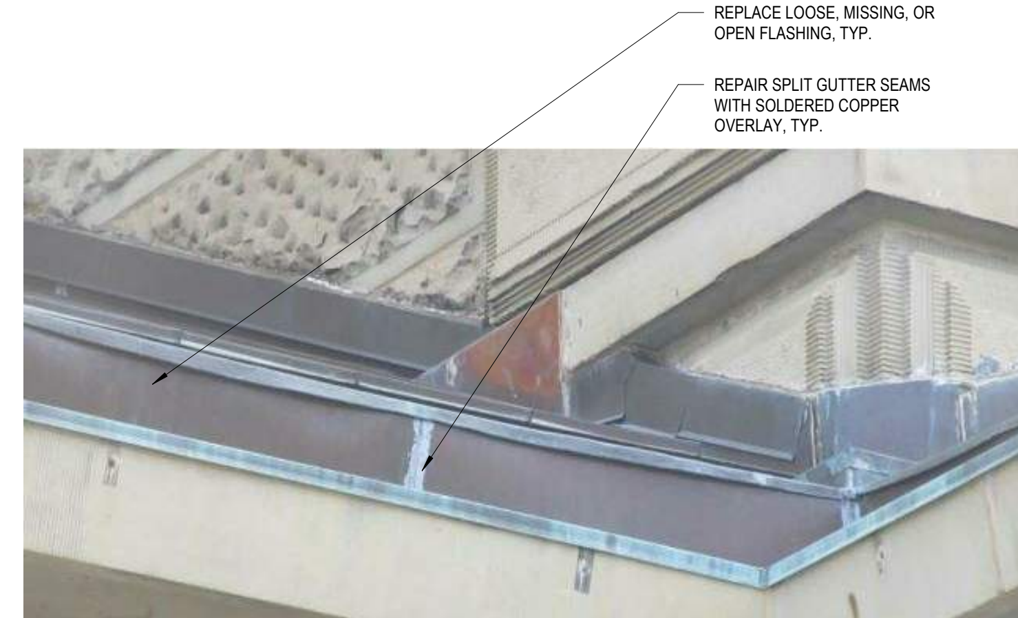
9 DETAIL @ ROOF CORNER FLASHING 1 1/2" = 1'-0"
