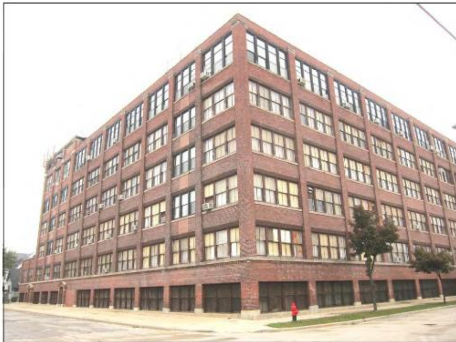
Image 11: West and south elevations, looking northeast (2013).
