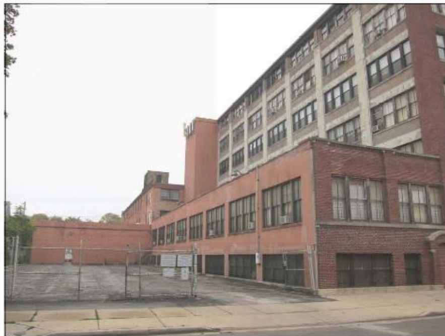
Image 19: North elevation, looking east (2013).
