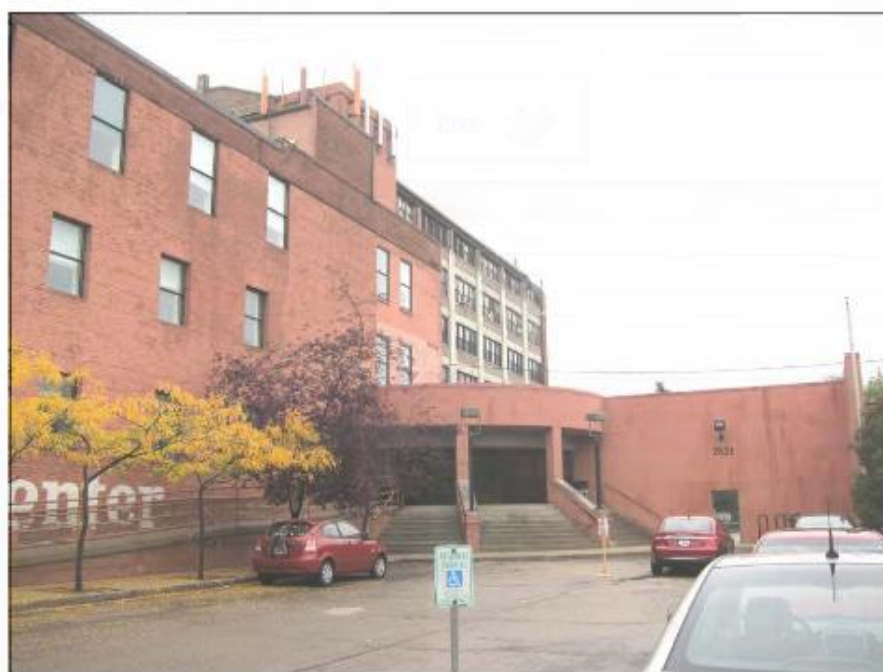
Image 18: North elevation, looking west (2013).
