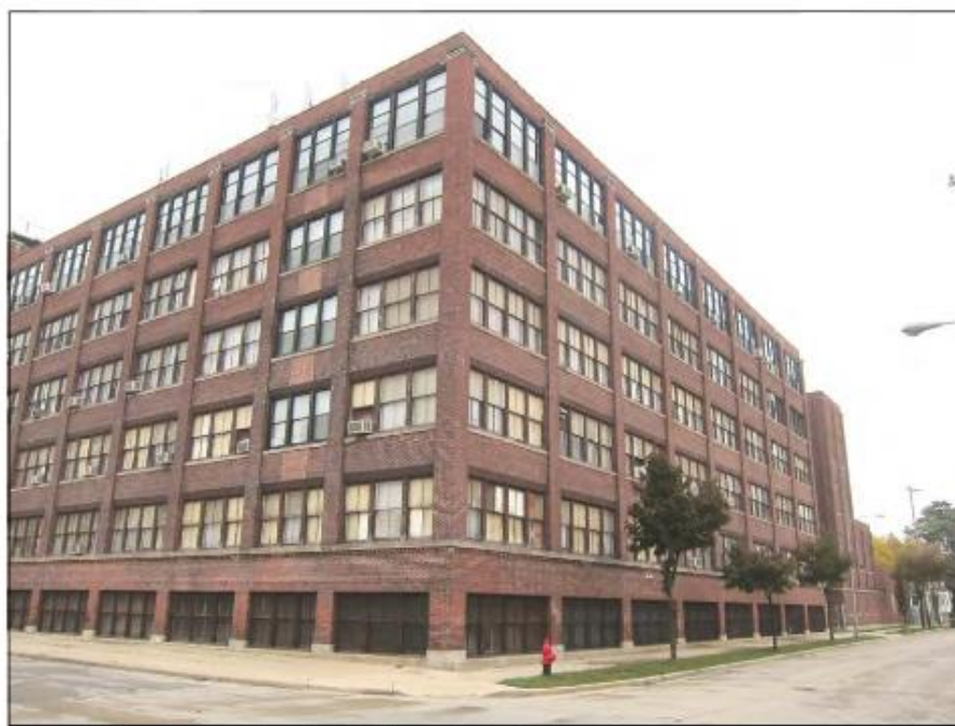
Image 12: West and south elevations, looking northeast (2013).
