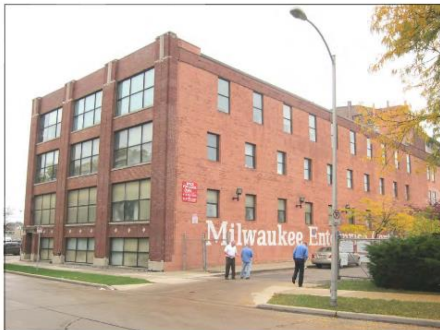
Image 17: East and north elevations, looking southwest (2013).
