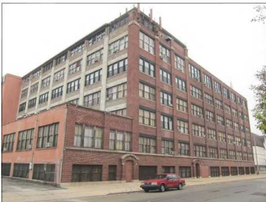
Image 20: North and west elevations, looking southeast (2013).
