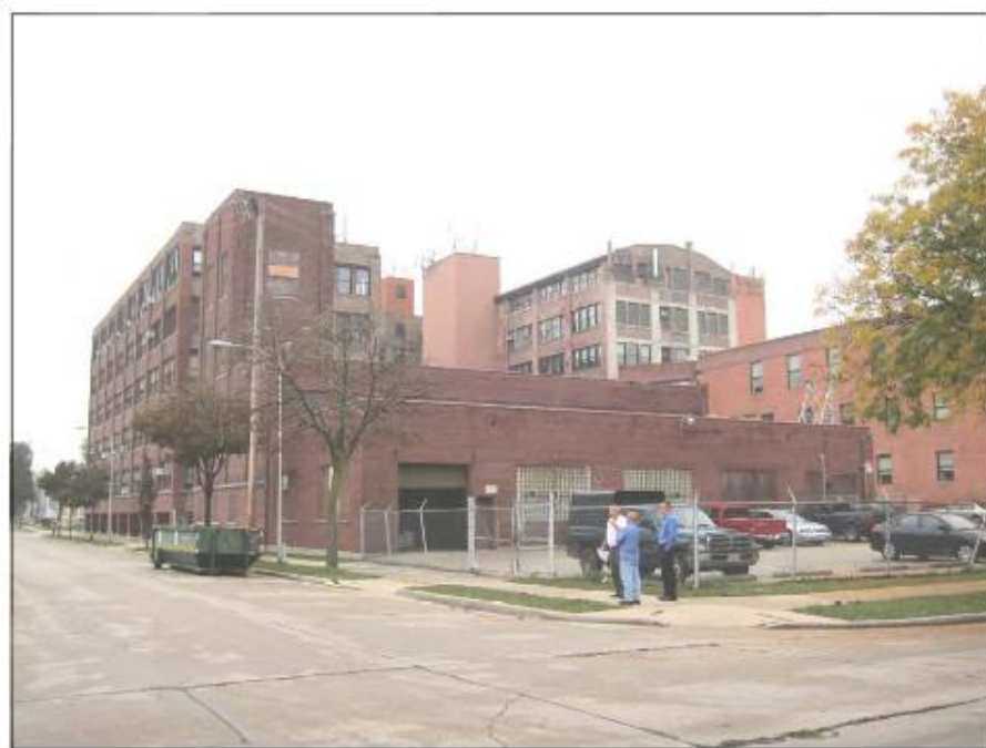
Image 14: South and east elevations, looking northwest (2013).
