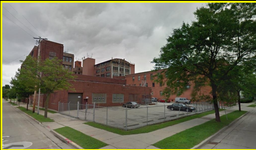
View of Site from W Hadley St and N 4 th St
