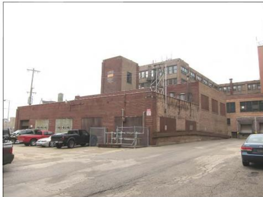
Image 15: East elevation, looking southwest (2013).
