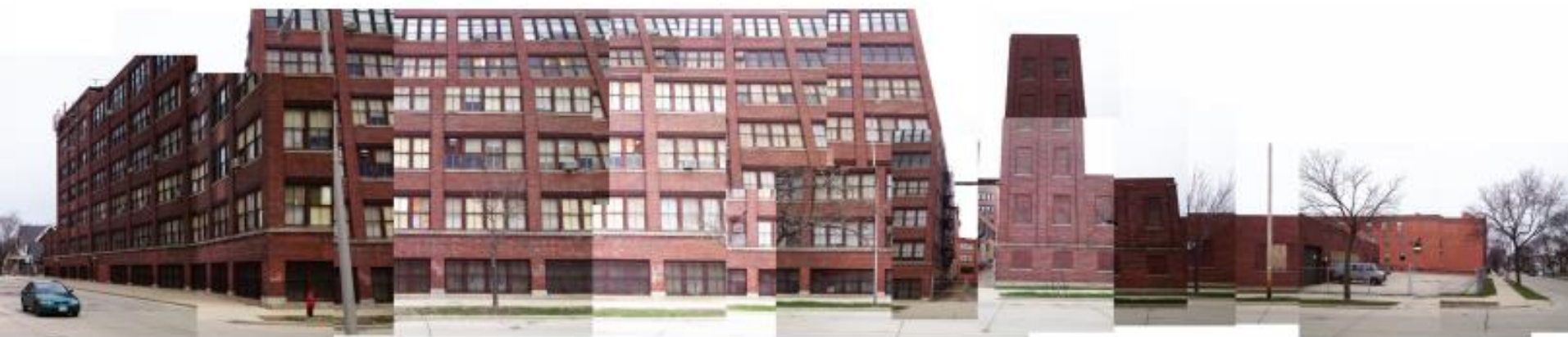
SOUTH ELEVATION FROM HADLEY
