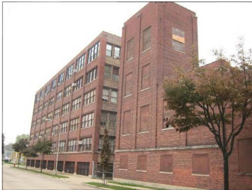
Image 13: South elevation, looking west (2013).
