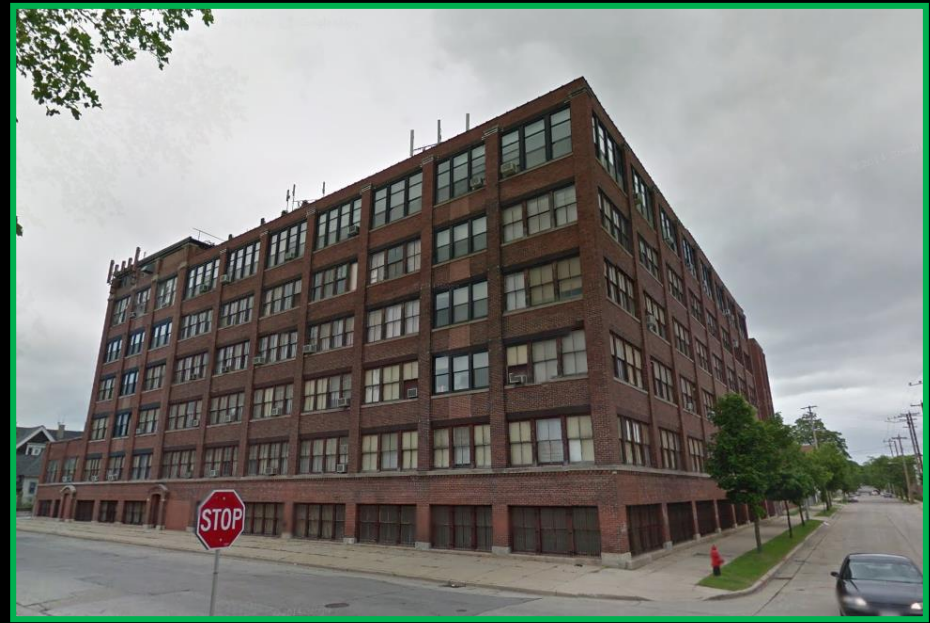
View of Site from W Hadley St and N 5 th St
