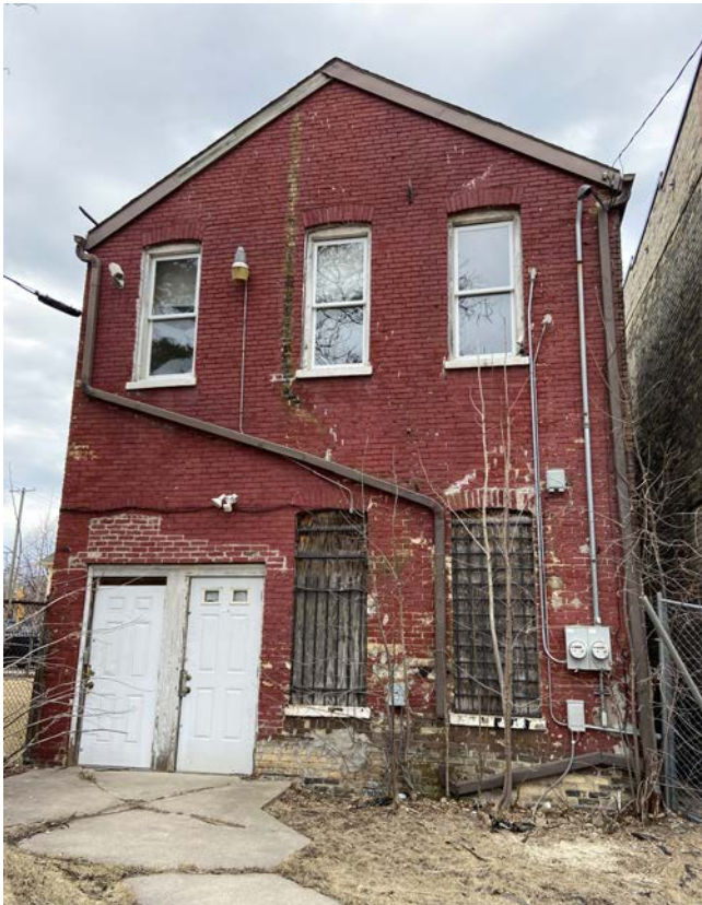
IMAGE 11: Rear area that will be reconfigured for ADA entrance, retaining wall, and new parking slab and walk.
