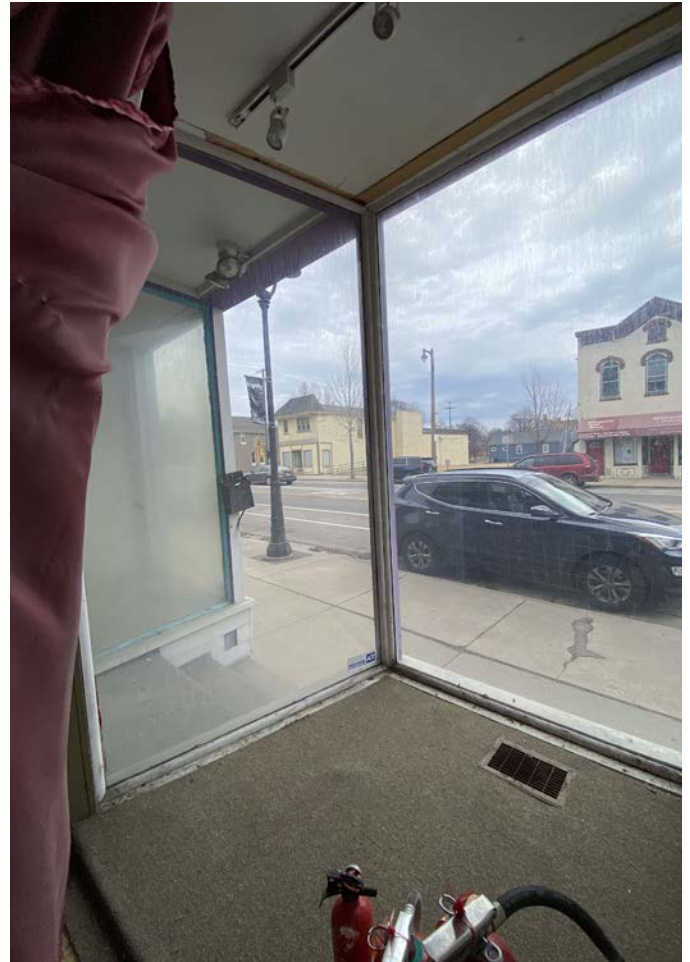
IMAGE 13: Interior side of existing storefront, south bay. New storefronts will preserve existing configuration and daylight openings and configuration.
