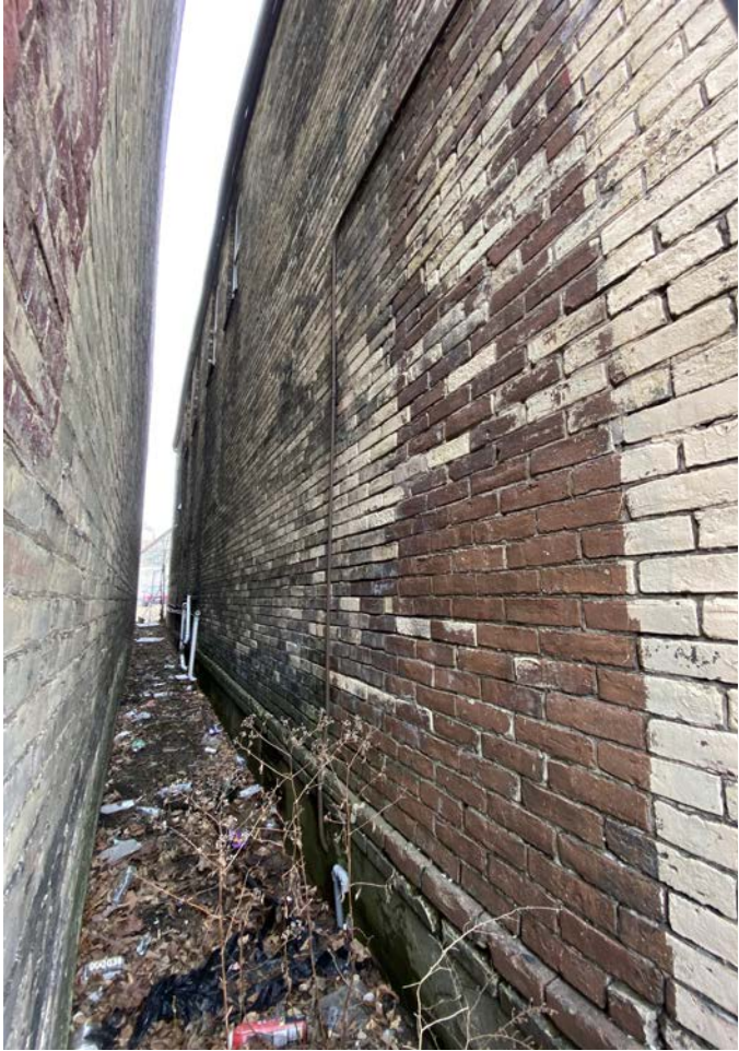
IMAGE 14: South elevation; here work is limited to masonry repairs and flashing at windows as described in the Scope Narrative.
