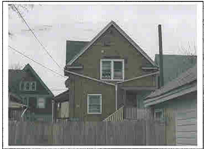
1542 W. Mineral St. – Rear View
