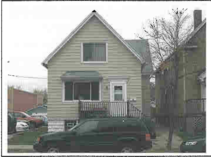
1546 W. Mineral St. – Front View
