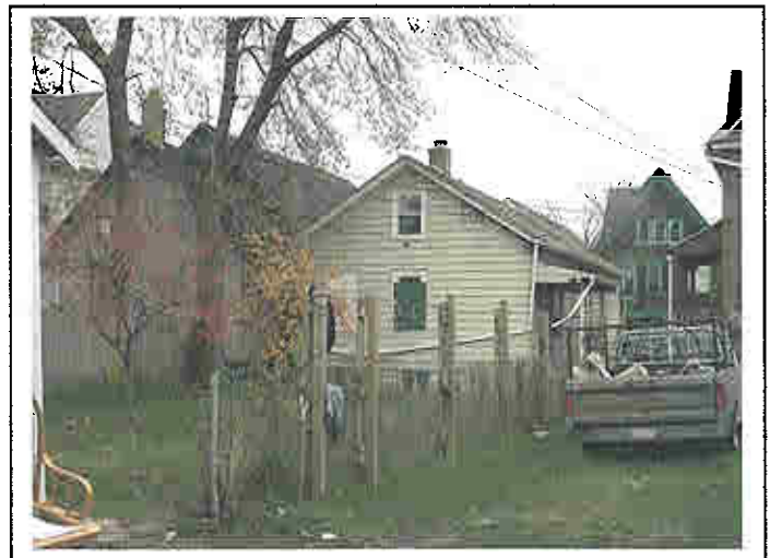
1540 W. Mineral St. – Rear View
