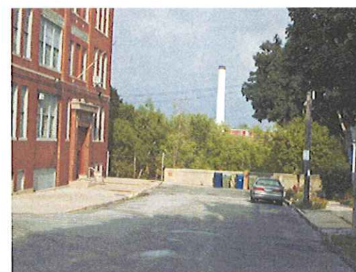
MEINECKE AVENUE LOOKING WEST
