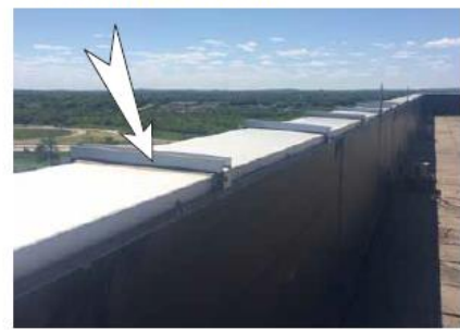
Fabricate new brackets & wireways
