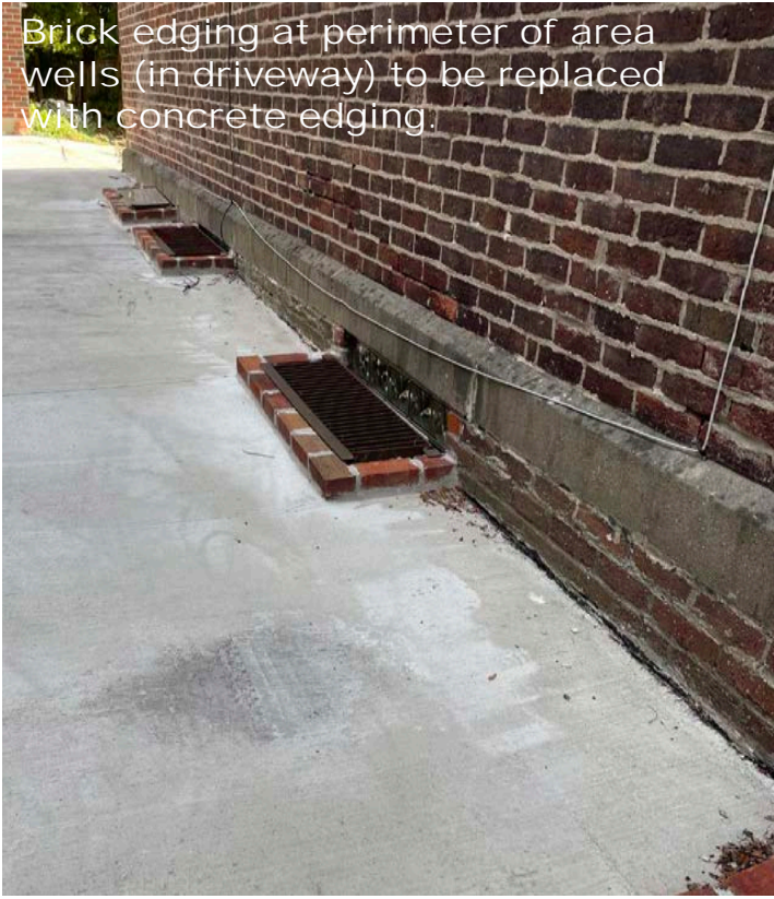
Concrete driveway to be regraded and replaced.
