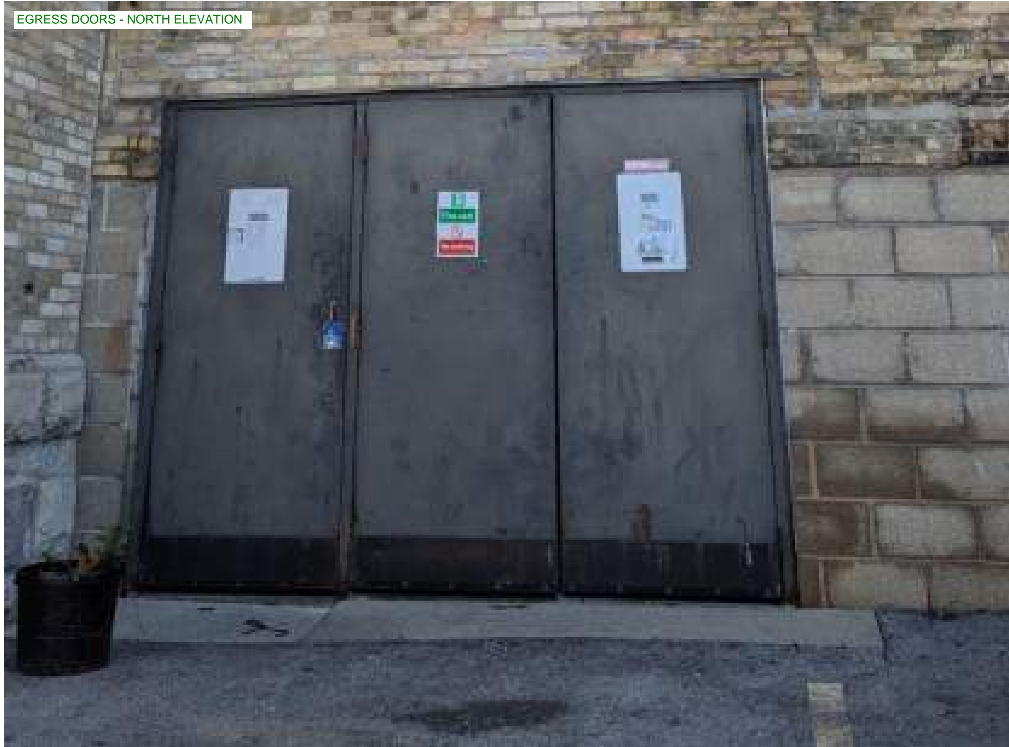
Non-original metal doors, in non-original opening to be replaced with new metal single panel doors. Doors and frames to be painted cream to match adjacent historic brick
