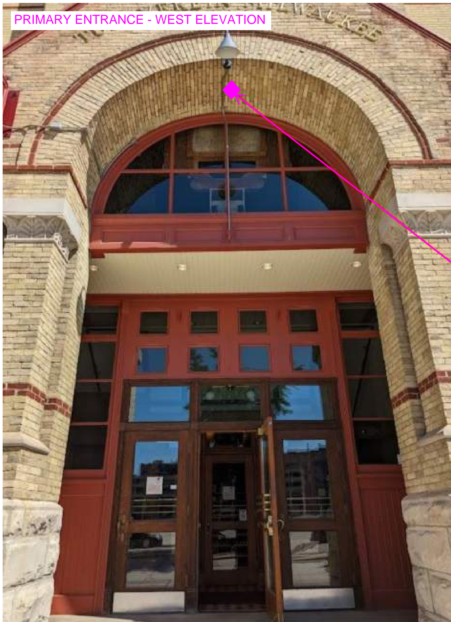
Surface Mounted Dome Camera. Paint white enclosure to match cream city brick color
