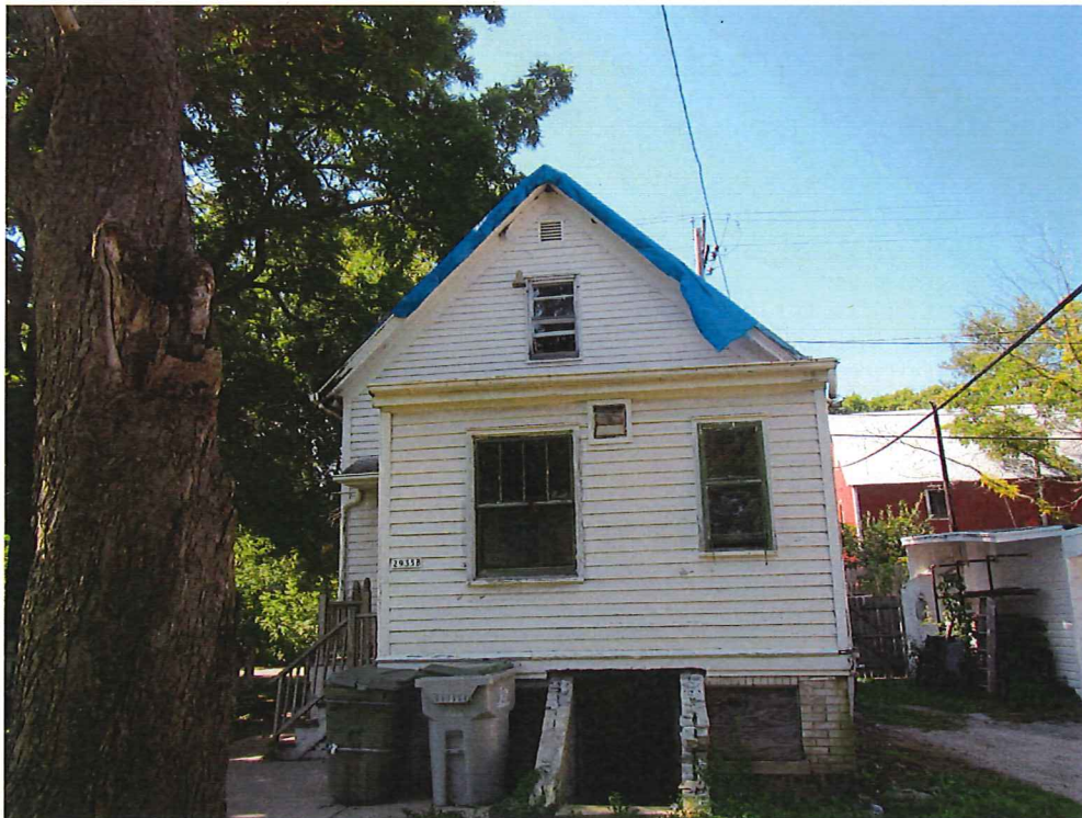
2935 North Richards – Rear House
