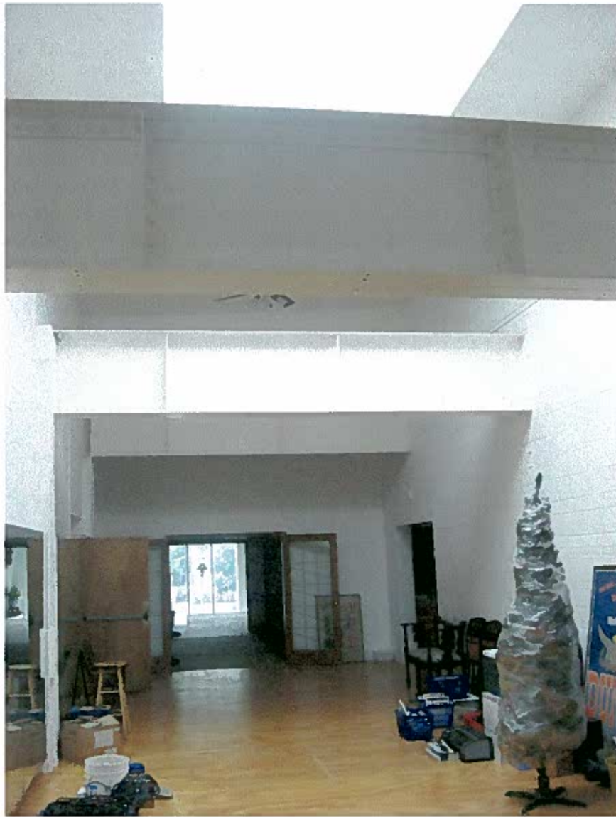
Existing second level space; floor to be removed for double height space. Some office and accessory space on remaining second level overlooking double height space. Space to be remodeled per construction plans.
