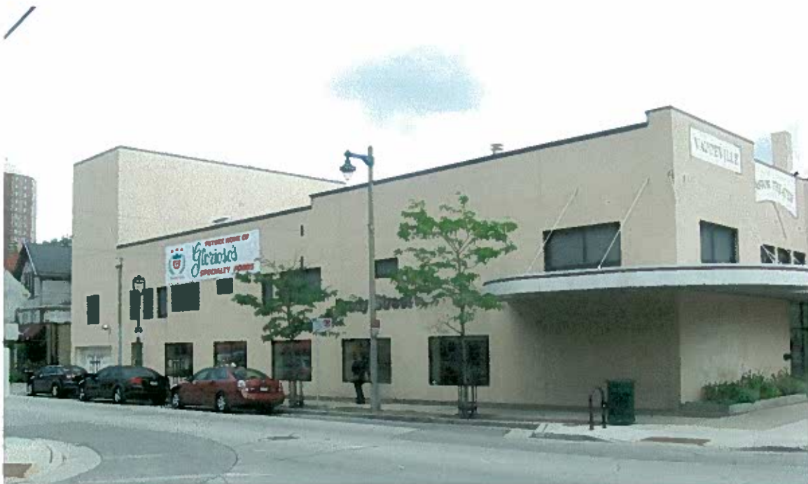
Existing building: Brady Street elevation. Building to be modified as shown on exterior elevation renderings including new cornice and trim board, signage, lighting, paint over existing eifs. Existing canopy to be modified as shown on exterior elevation renderings; canopy above main entrance kept and rewrapped with metal coping. New awnings with signage to be added to Brady Street sidewalk level windows as shown on exterior elevation renderings.
