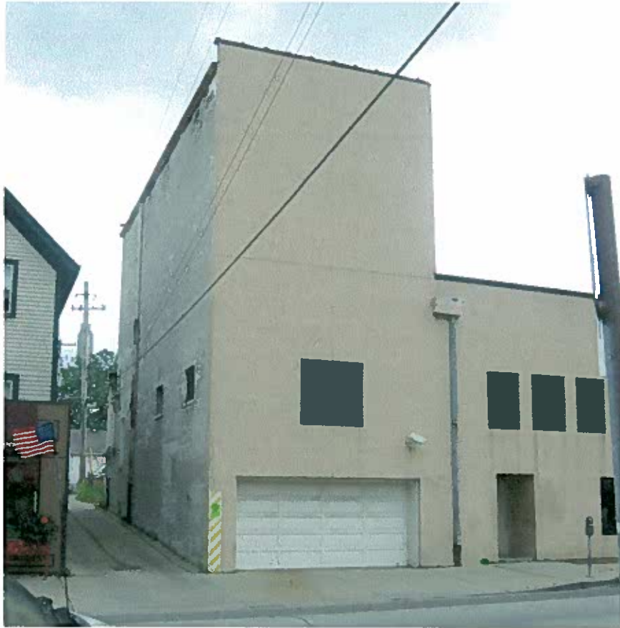
Existing building: Brady Street elevation. Building to be modified as shown on exterior elevation renderings including new cornice and trim board, signage, lighting, paint over existing eifs. Garage door to be replaced with fixed wood panel garage door.
