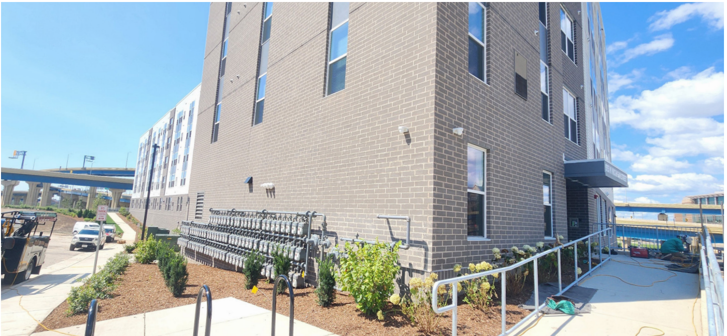
Outside progress as of summer 2024.
