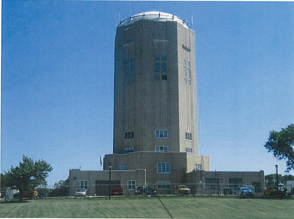
Fig. 2 EXISTING Elevation Looking East
