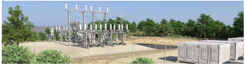
Figure 5 Constructed Substation Facility
