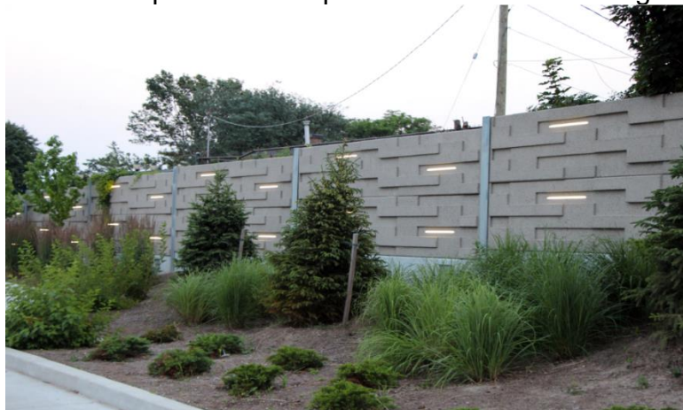
Figure 8 Example of Exterior Sound Barrier Wall
