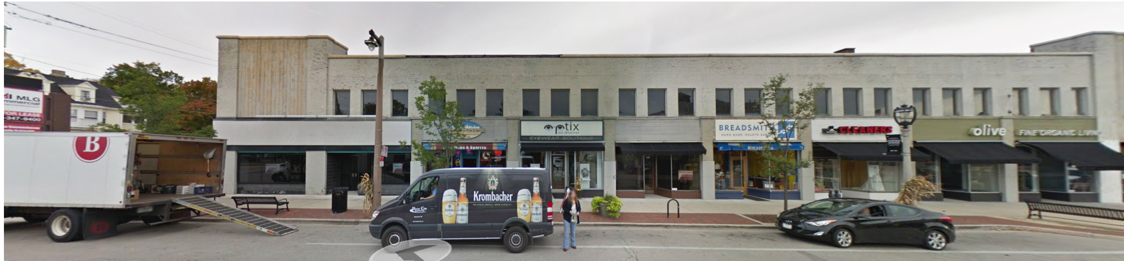
Existing Street Facade
