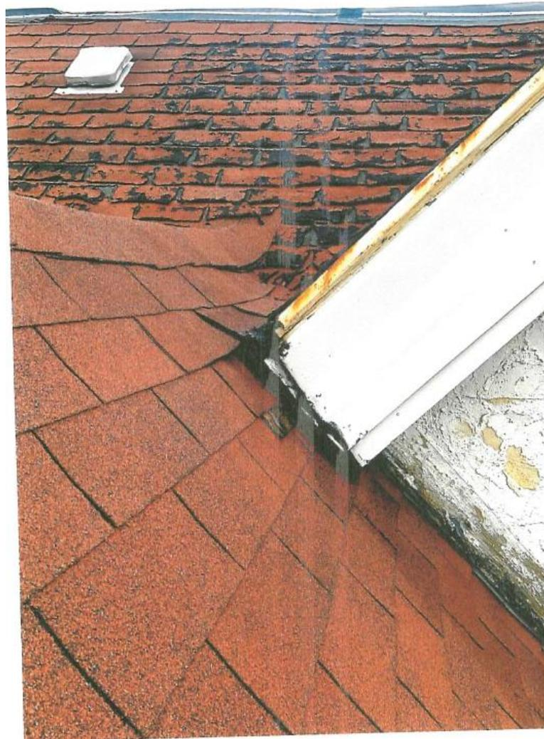
Valleys **must** be metal, **NO** interweaving of shingles (as is shown above is present condition)
