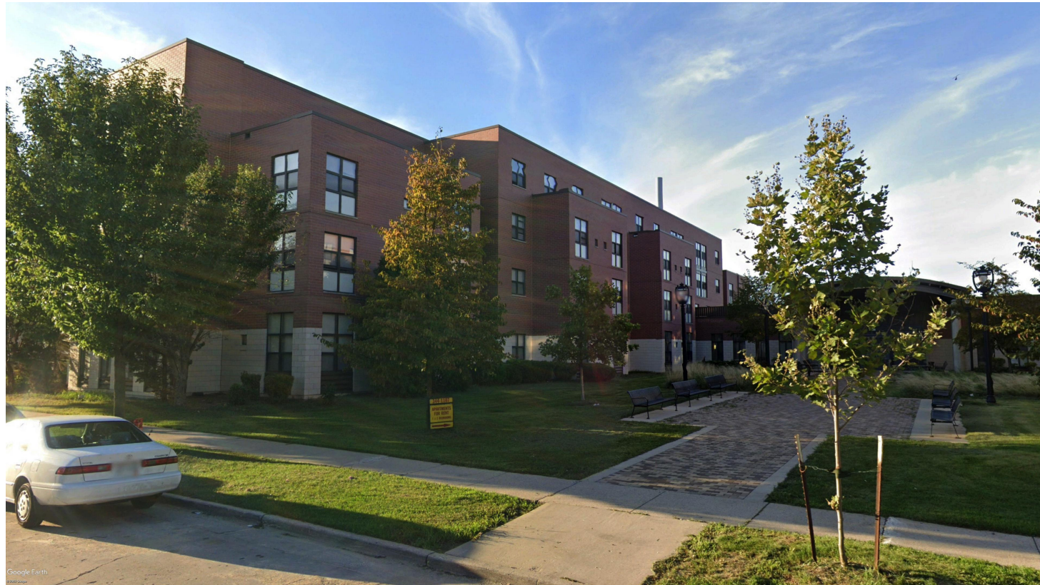
EXISTING WEST WING
