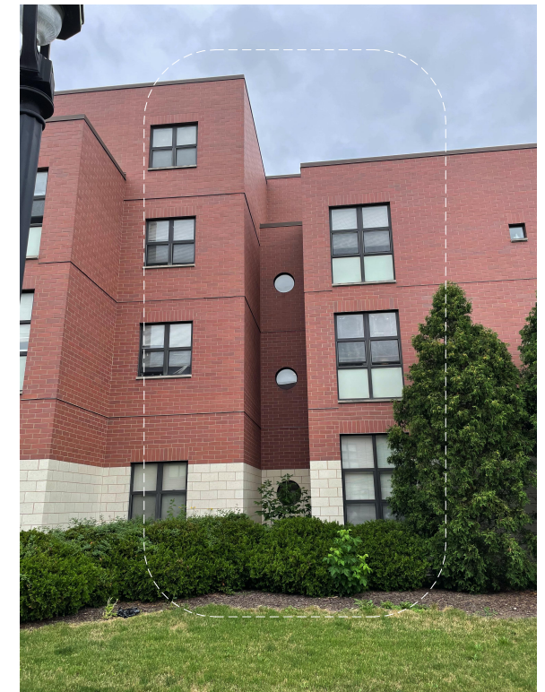
EAST WING - AREA OF WORK
