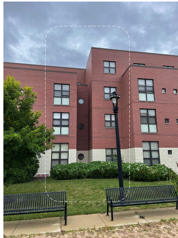
WEST WING - AREA OF WORK
