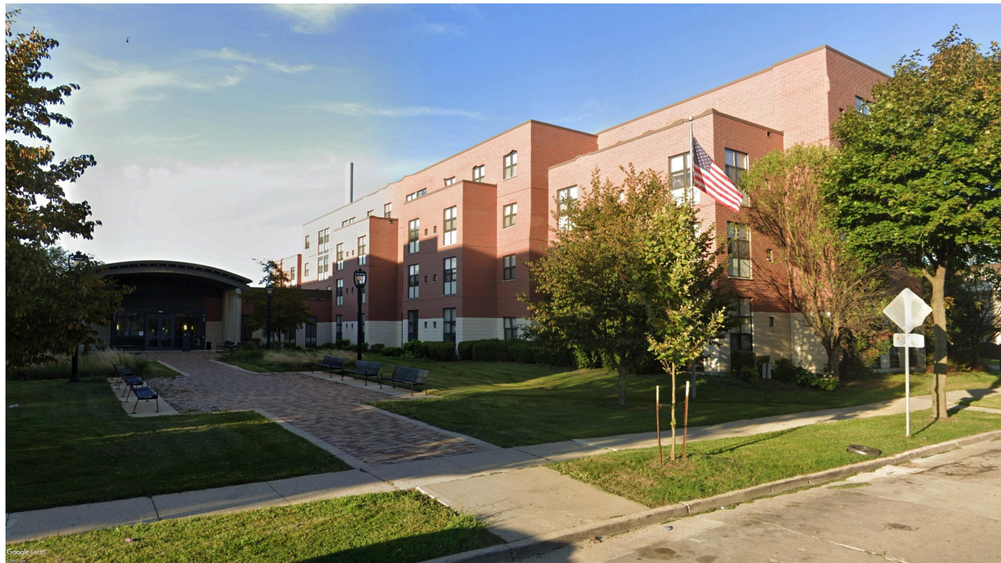
EXISTING EAST WING
