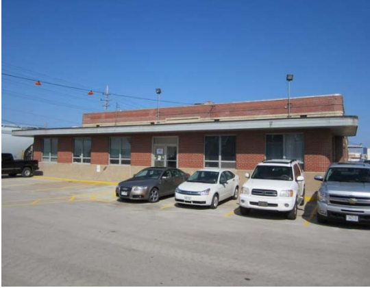
Brick and concrete at south elevation
