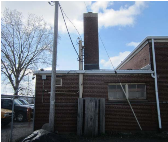
Gutters at north elevation
