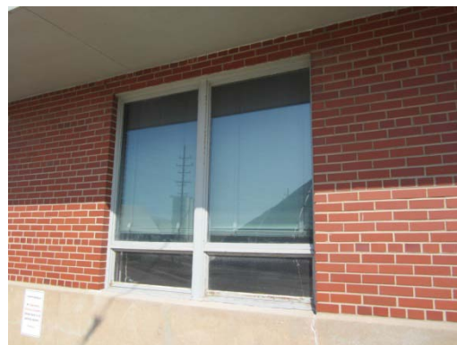
East elevation window possibly replaced
