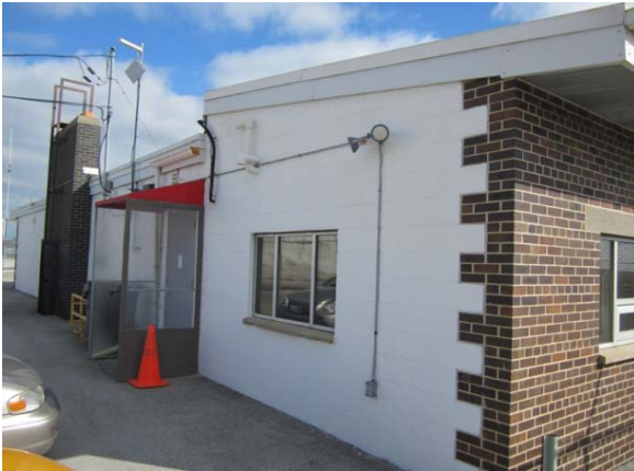
CMU and brick west elevation
