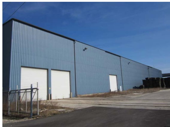
South building gutters & downspouts
