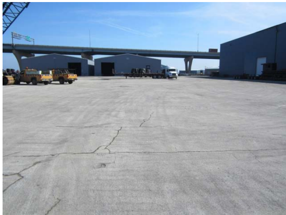
Parking lot overview
