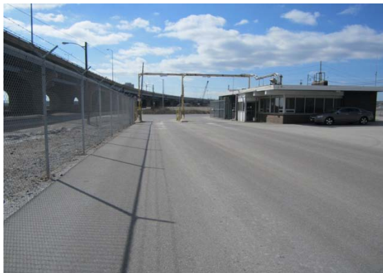
Entrance asphalt driveway overview
