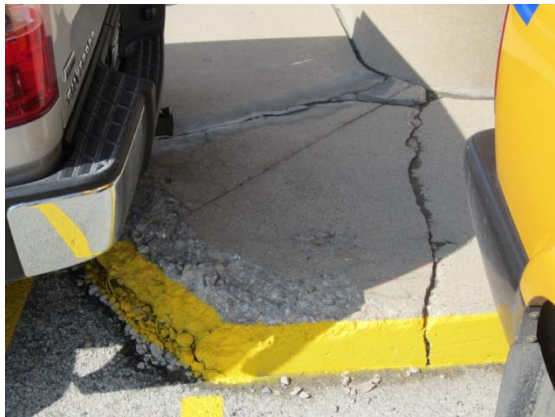
Cracked concrete
