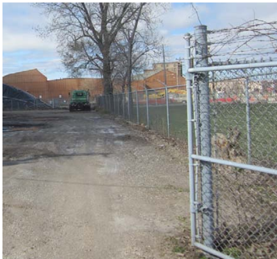
Fence at north perimeter
