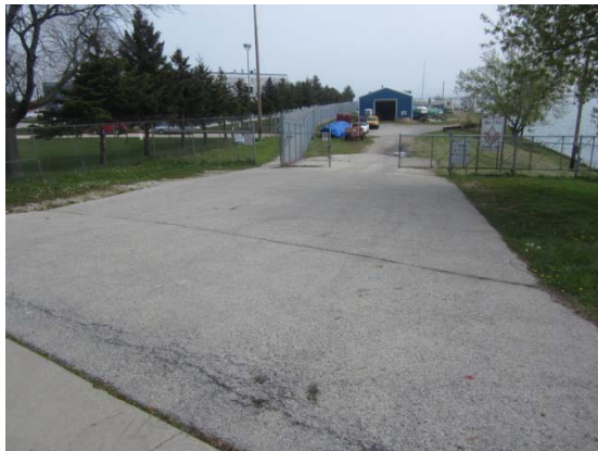
Entrance Asphalt driveway overview
