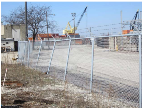
Chain link fence south
