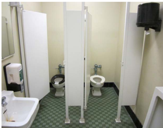
Men's room toilets, partitions
