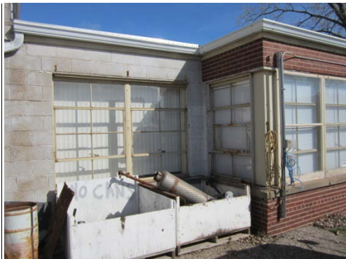
South elevation windows
