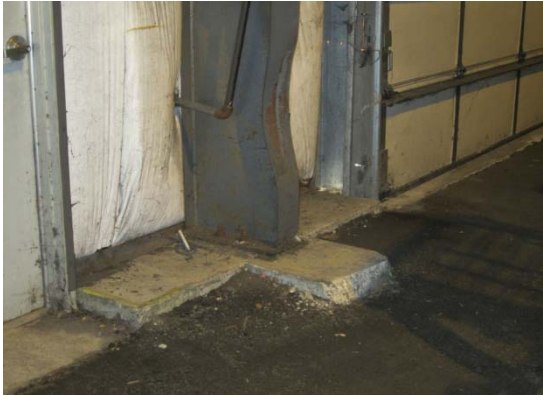
Pavement overlay at building perimeter
