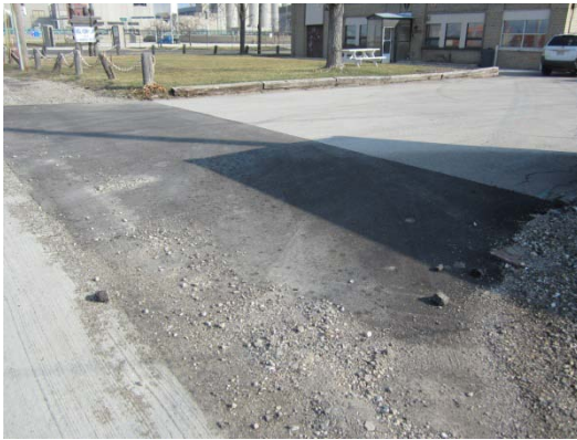
Recently replaced driveway apron
