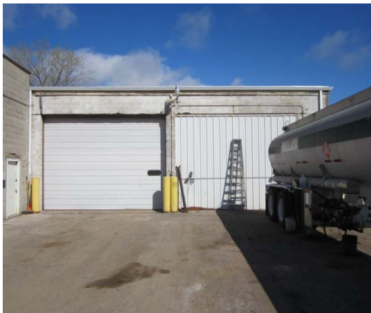
South elevation overhead garage door
