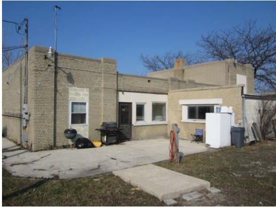
East elevation cracking asphalt pavement
