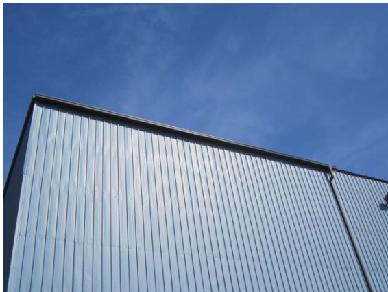
Gutters and downspout
