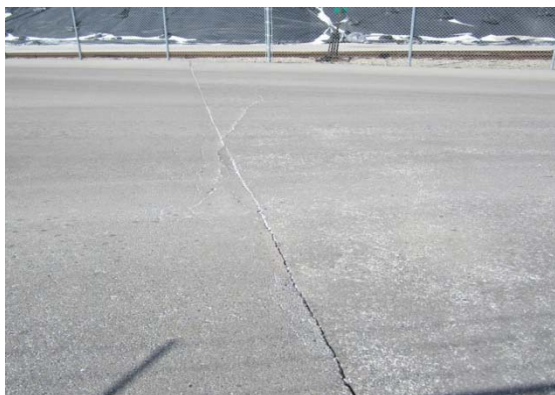
Traverse cracking
