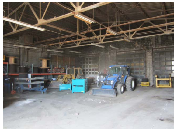
Light fixtures at Port garage
