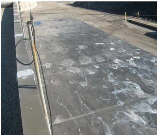
Roof-3 elevation view
