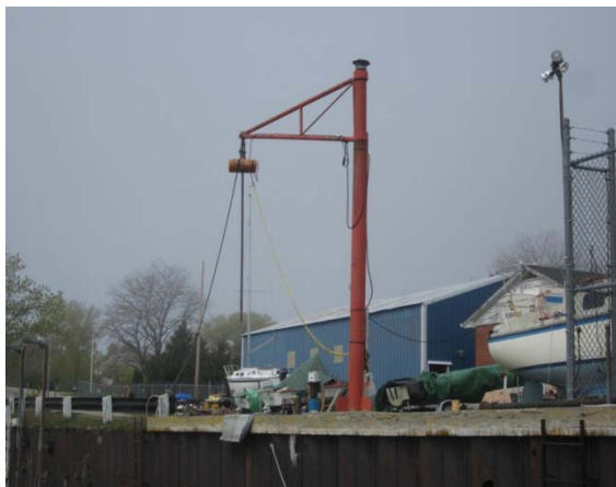
Boat Crane east elevation
