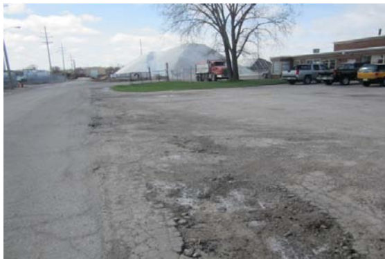
Entrance Asphalt driveway overview
