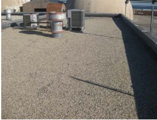
Roof-2 elevation view
