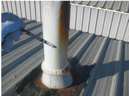
Rusted flashing
