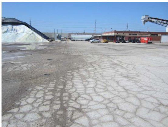
Alligator cracks
