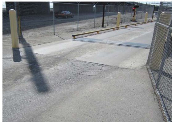
Cracked pavement
