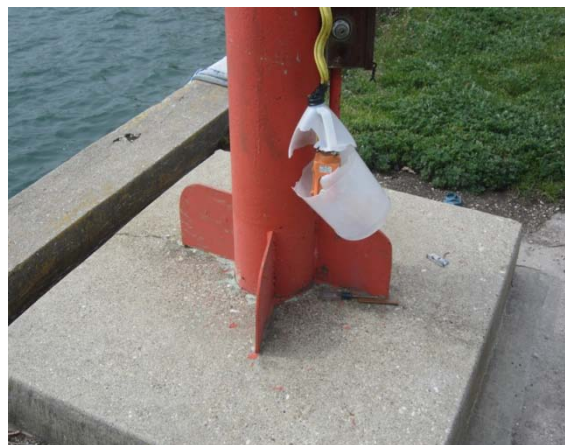
Cracked foundation
