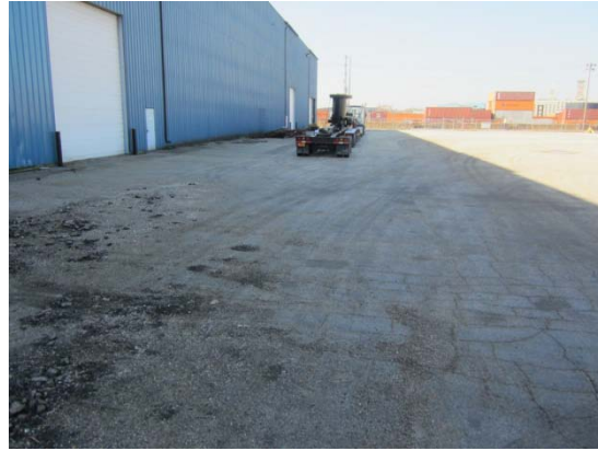
Failed pavement
