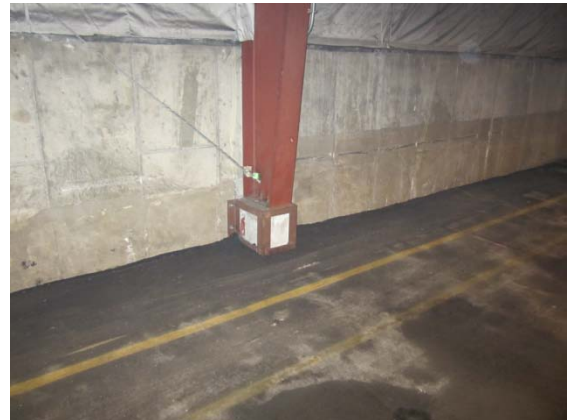
Pavement overlay at building perimeter
