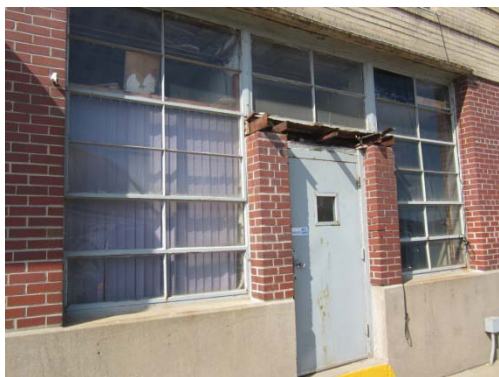
Window system at east elevation
