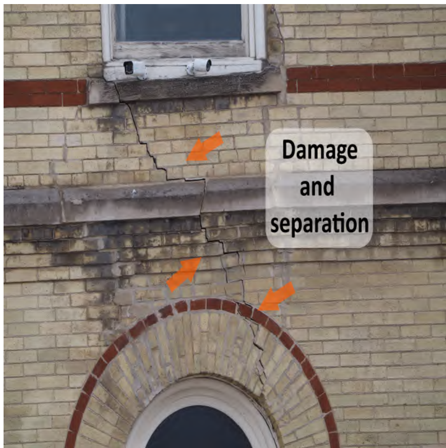
-West facade below second floor window
