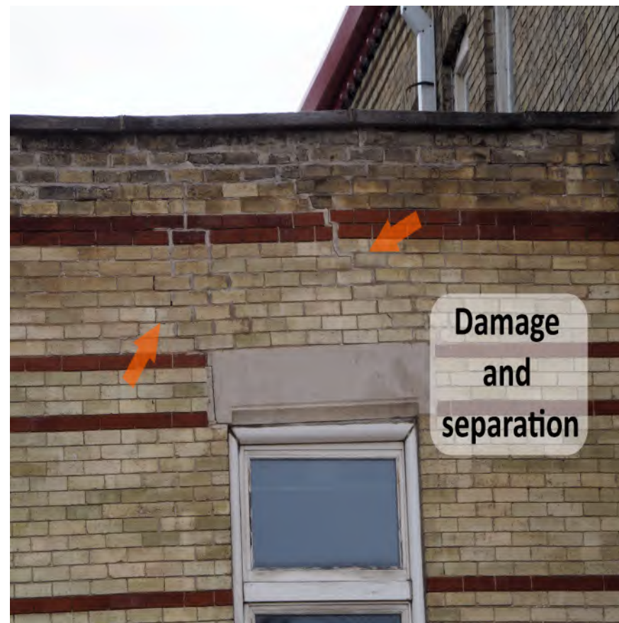
-West facade above second floor window
