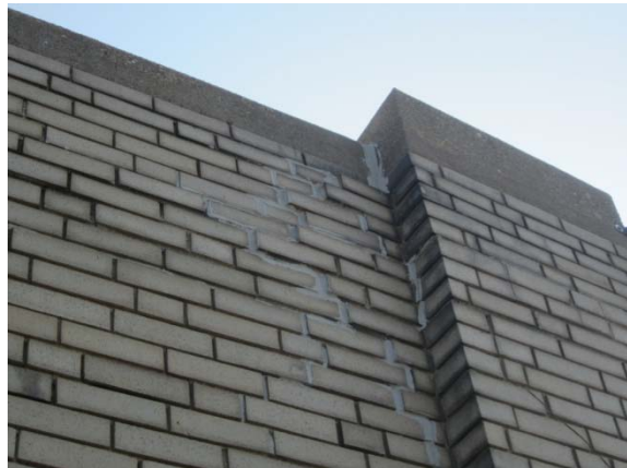
Sealant (not mortar) repair
