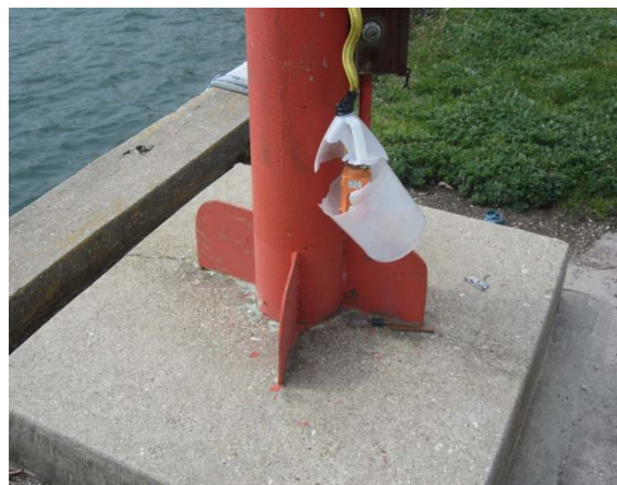
Cracked foundation
