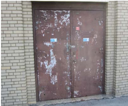
West mechanical room doors
