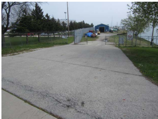
Entrance Asphalt driveway overview
