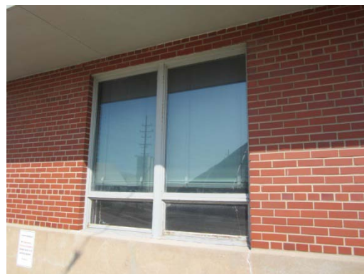
East elevation window possibly replaced
