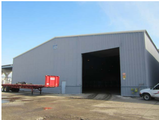
West overhead door with high use
