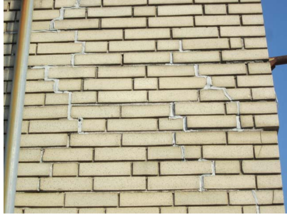
Sealant (not mortar) repair at masonry
