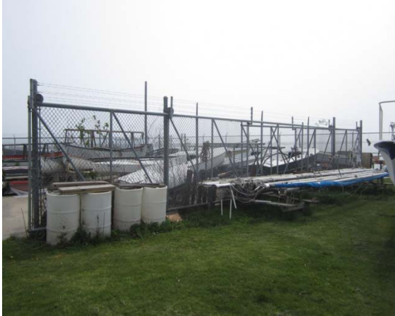
East elevation chain link sliding gate
