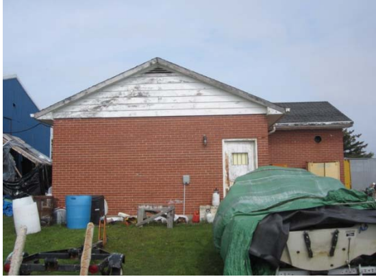
Brick from the east elevation
