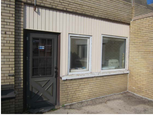
East elevation windows – replaced (not original)
