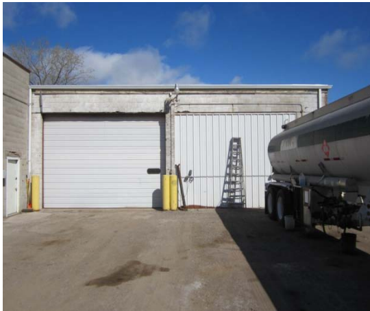
South elevation overhead garage door
