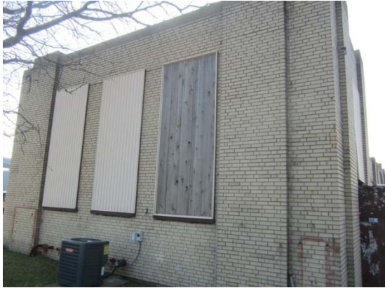
Boarded Brick windows north elevation
