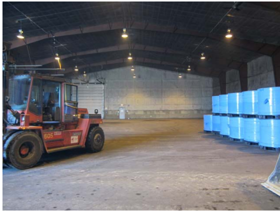
Interior photograph – note light fixtures
