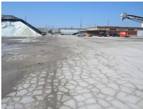
Alligator cracks
