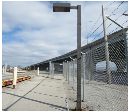
Light fixture with
