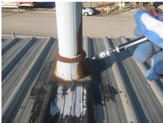
Rusted flashing
