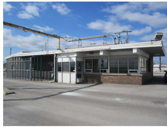
East/north elevations include highest concentration of windows/doors
