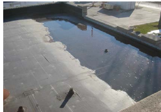
Ponding water R-1, drain stopped up
