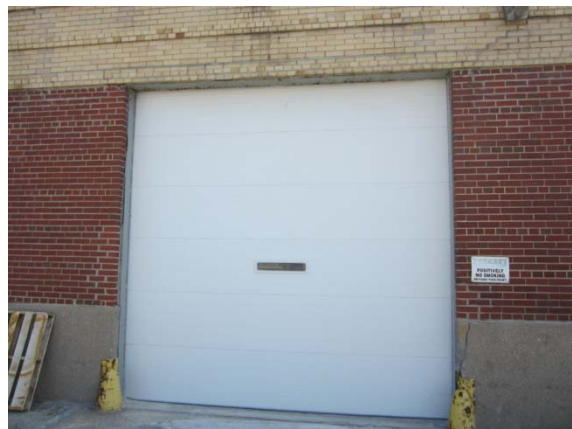
West elevation garage door recently replaced
