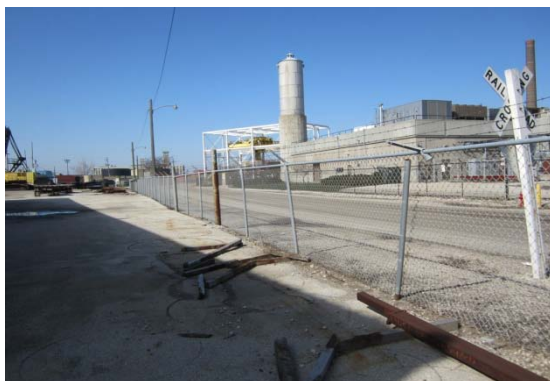
North chain link fence
