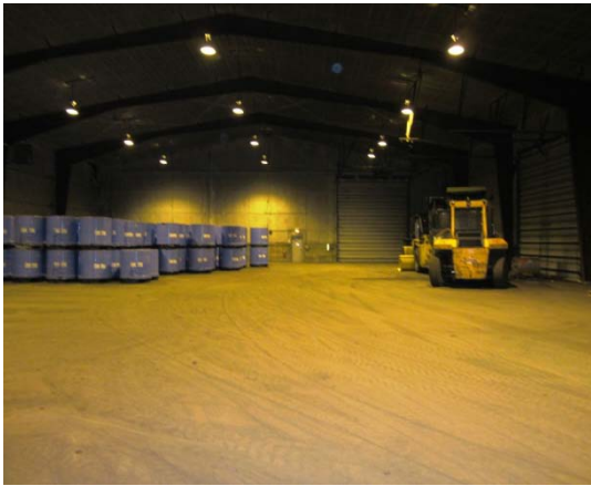
Interior photograph – note light fixtures
