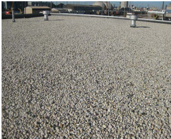
Roof-1 elevation view
