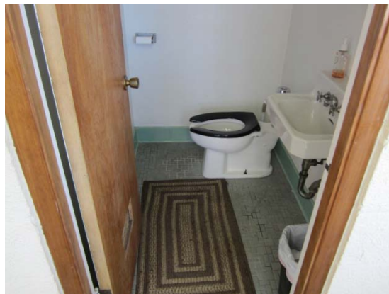
Rest room finishes
