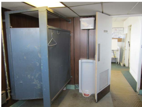
Rest room finishes
