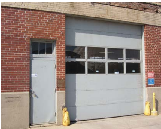
East elevation overhead garage door
