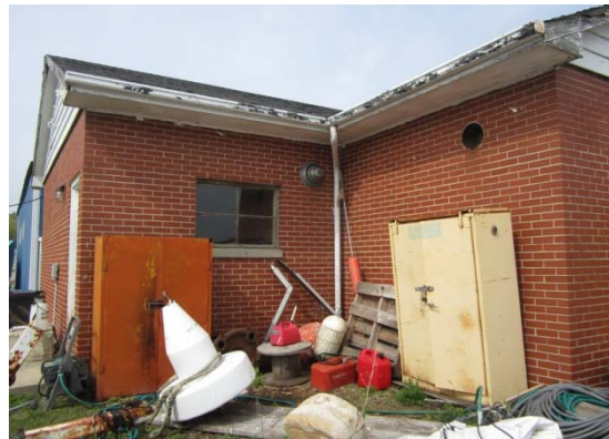
Gutters and downspout
