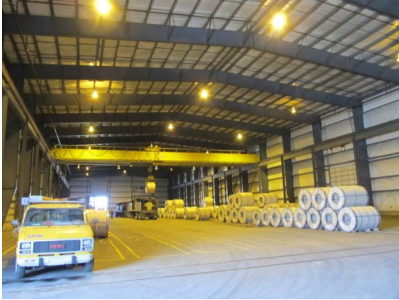
Overhead crane service
