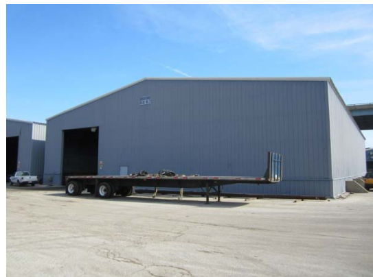
West overhead door with high usage
