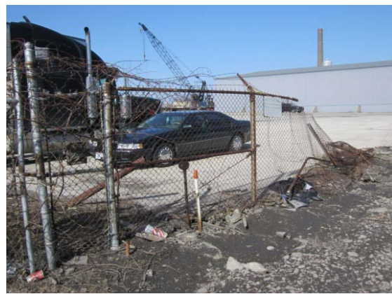
Failed fence at east
