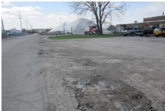
Entrance Asphalt driveway overview
