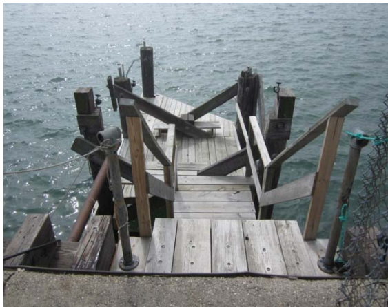
Wooden Pier east elevation
