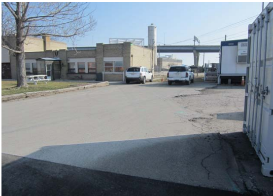
Entrance Asphalt driveway overview
