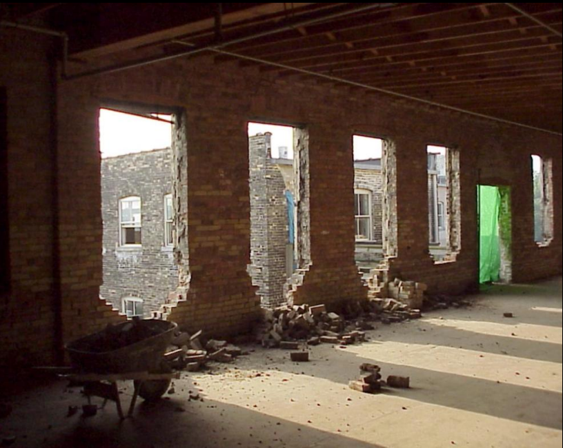
1236 W. Pierce St. - IH to IM During Restoration
