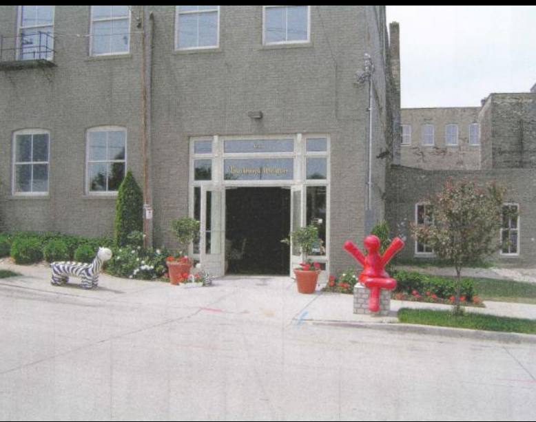
1236 W. Pierce St. - IH to IM After Restoration
