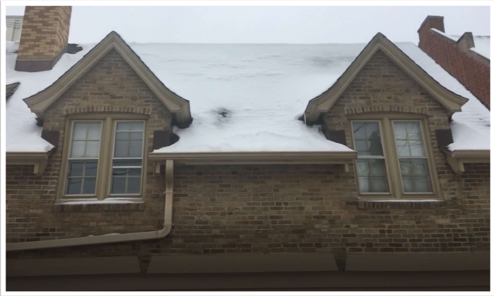
Figure 7. Some of storm/screen combinations to be replaced on east elevation.
