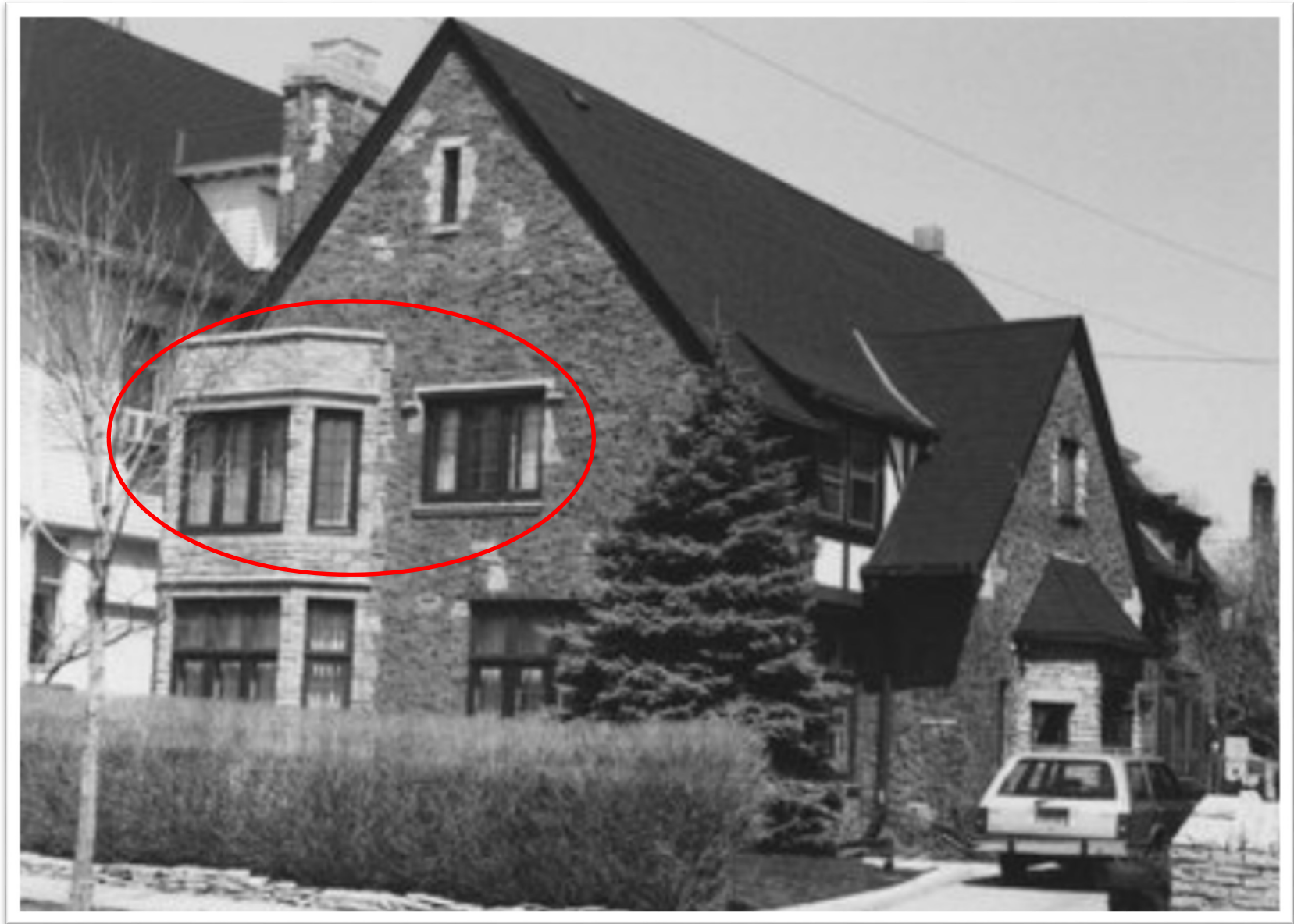
Figure 3. South and east elevations circa 1970's-80's, showing the presumed original windows that were later replaced with Pella casements.
