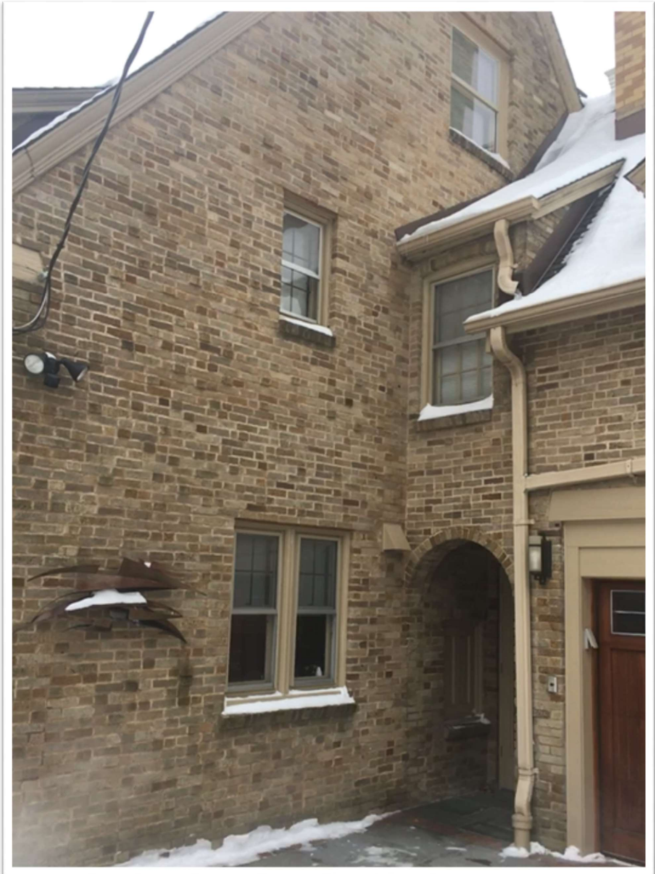
Figure 9. Some of storm/screen combinations to be replaced on north and east elevations.
