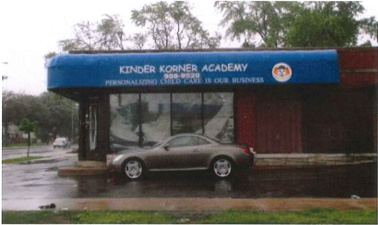
6003-05 West Villard Avenue
