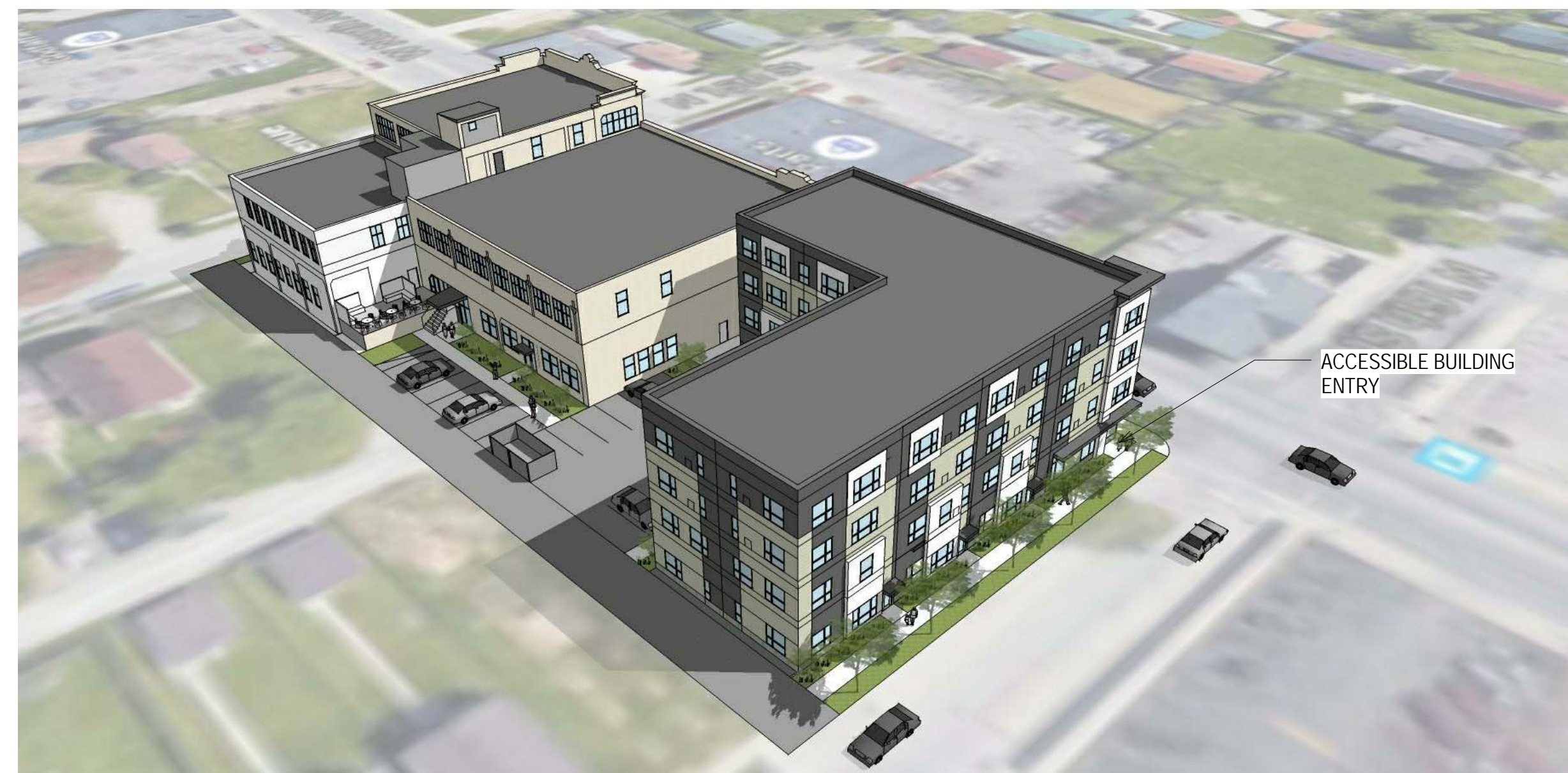
BIRDSEYE VIEW - TOWARD THE SOUTHEAST
