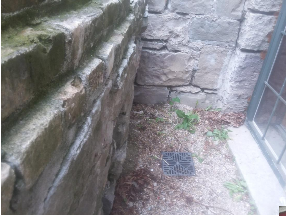
Area to be rebuilt.
