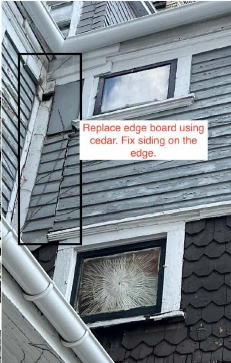
Replace edge board using cedar. Fix siding on the edge.
