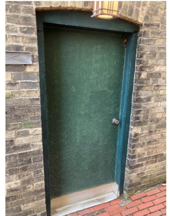
Lower level Side door to be opened up. (North Face)
