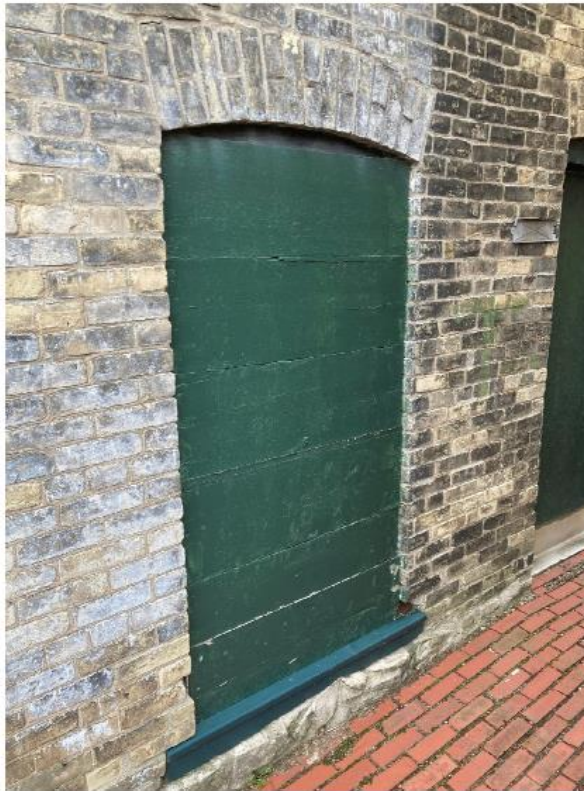
Lower Level Window to be opened up (North Face)
