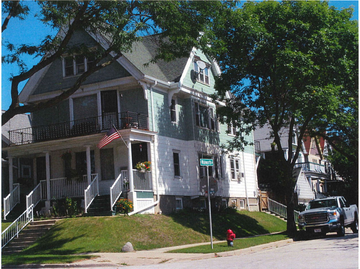
2344 North Humboldt Ave
