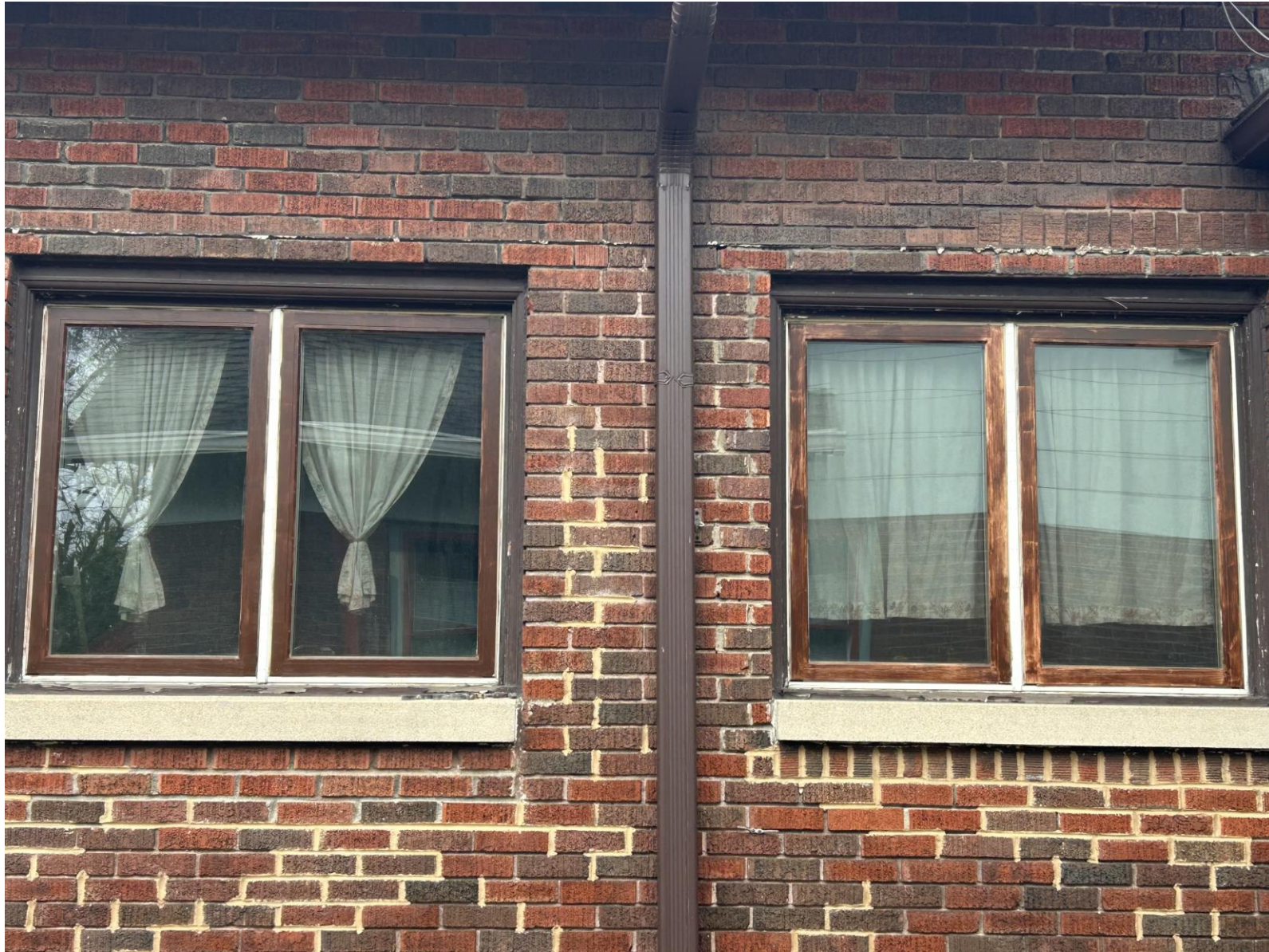
New casement windows in November 2025. Painting in progress.
